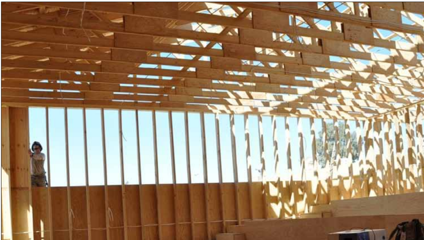
Second Lt. Jacob Della Pia, of Manistee, Mich., applies sheeting to the side of the new Command Division Operations Center at Contingency Operating Location Deason. The 101st Engineer Battalion has helped 17th Iraqi Army engineers become a self-sufficient asset to their division by teaching them some basic carpentry skills.
