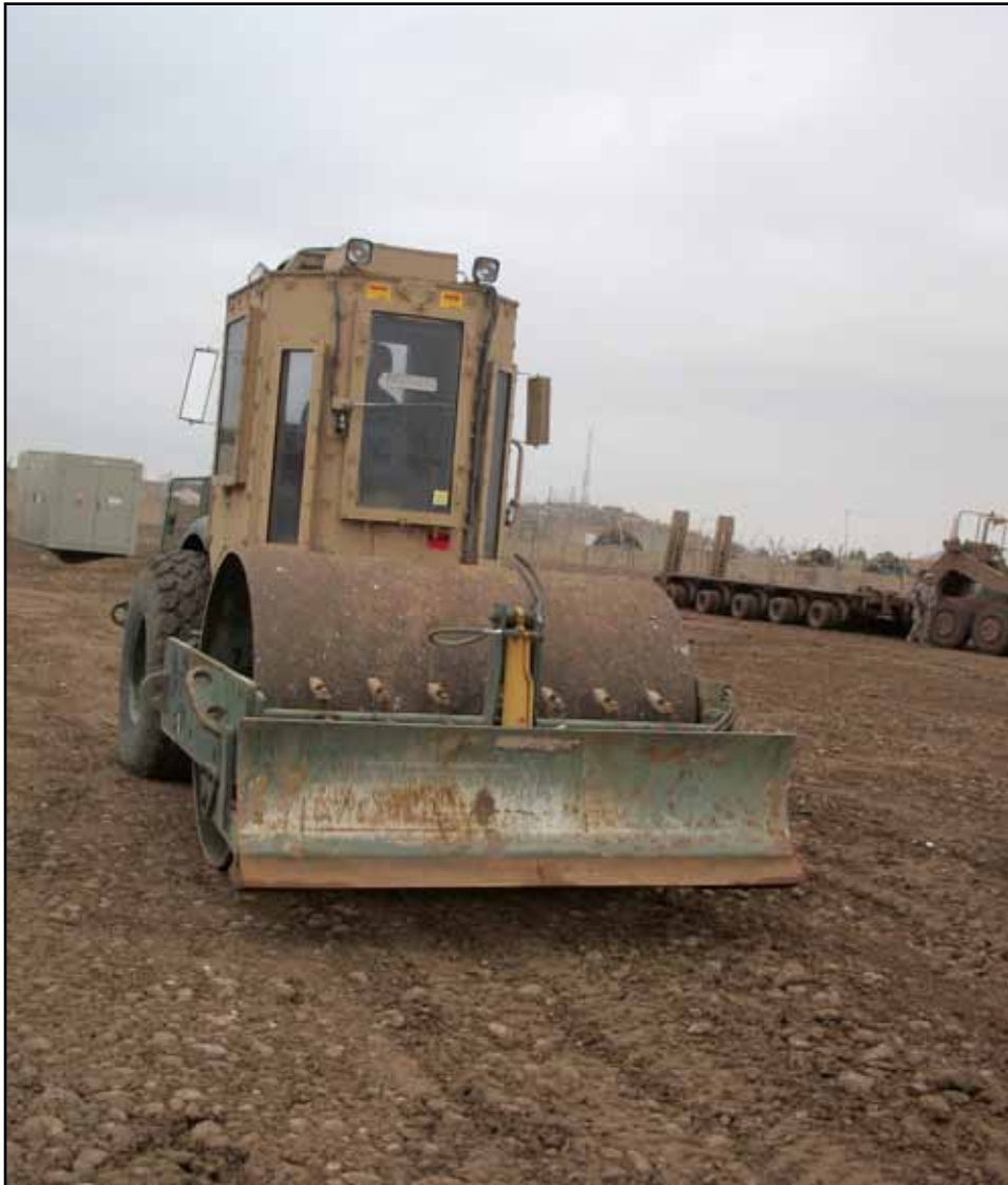
Spc. John Broccardo, 317th Engineer Company, operates a roller, putting finishing touches to a portion of the Mobile Redistribution Team's yard that will help mitigate the mud problem in the parking lot.
