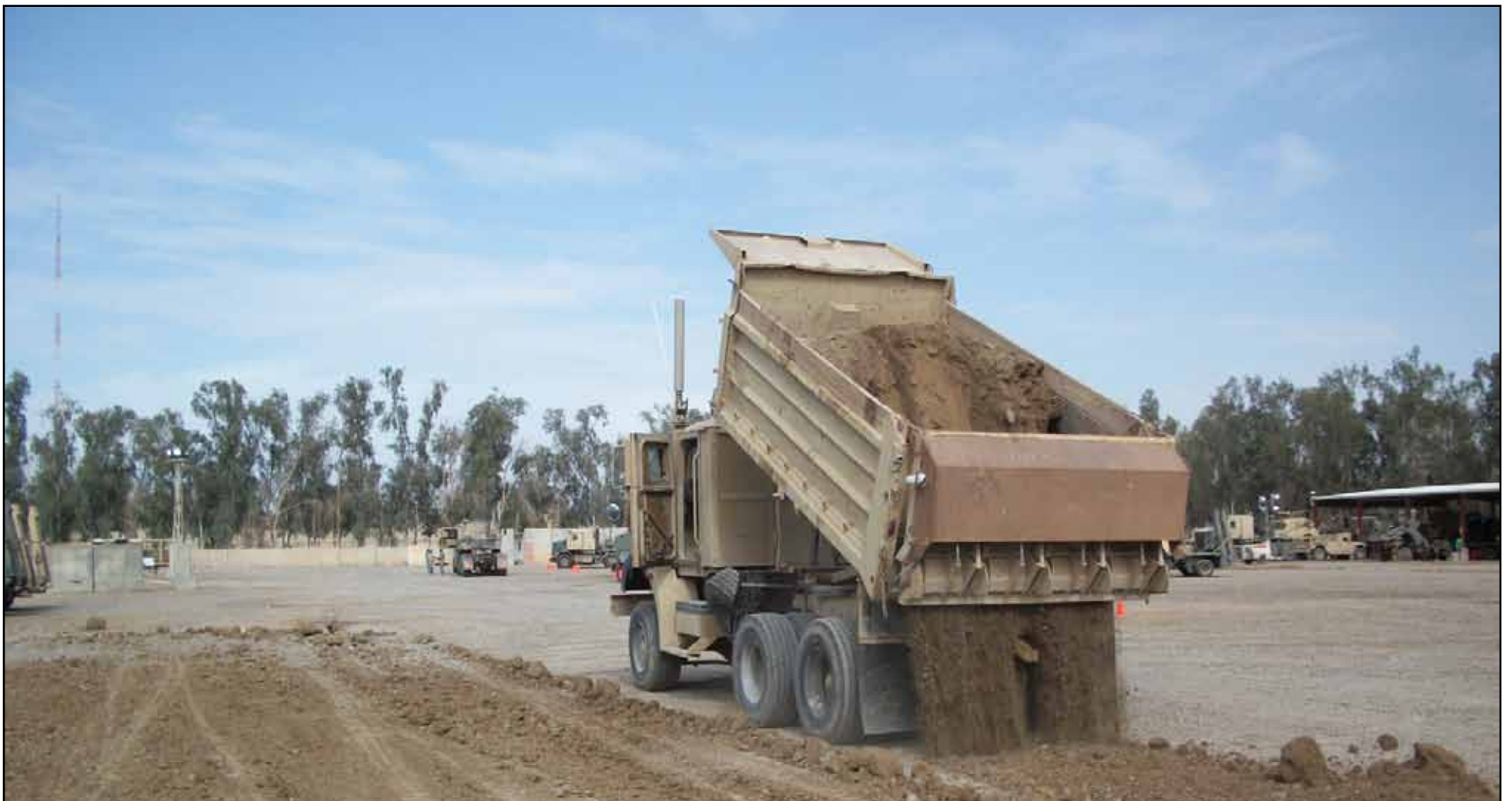
BAGHDAD — Spc. Robert Smith, 317th Engineer Company, empties a load of gravel at the Mobile Redistribution Team's yard at Victory Base Complex March 12. The engineers have been working at the MRT yard to improve the surface and drainage, which will mitigate the current mud and flooding problems.
