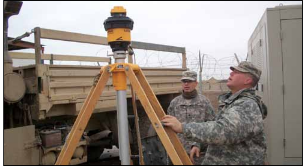
Spc. Bret Harmon (right) and Sgt. Brian Guzman (left), 317th Engineer Company, are setting up a laser level at the Mobile Redistribution Team, the device is used to ensure surface repairs are as smooth as possible.
