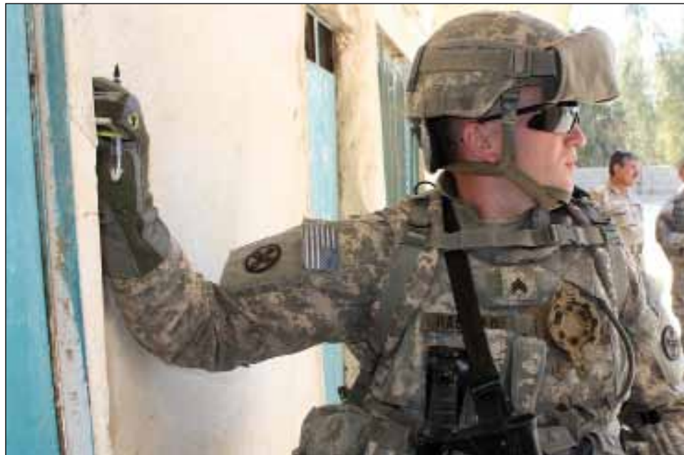
In an effort to determine the level of repairs needed, Sgt. Andrew Rasfeld uses a Robyi TEK4 professional laser distance measure at a school in Baghdad.
