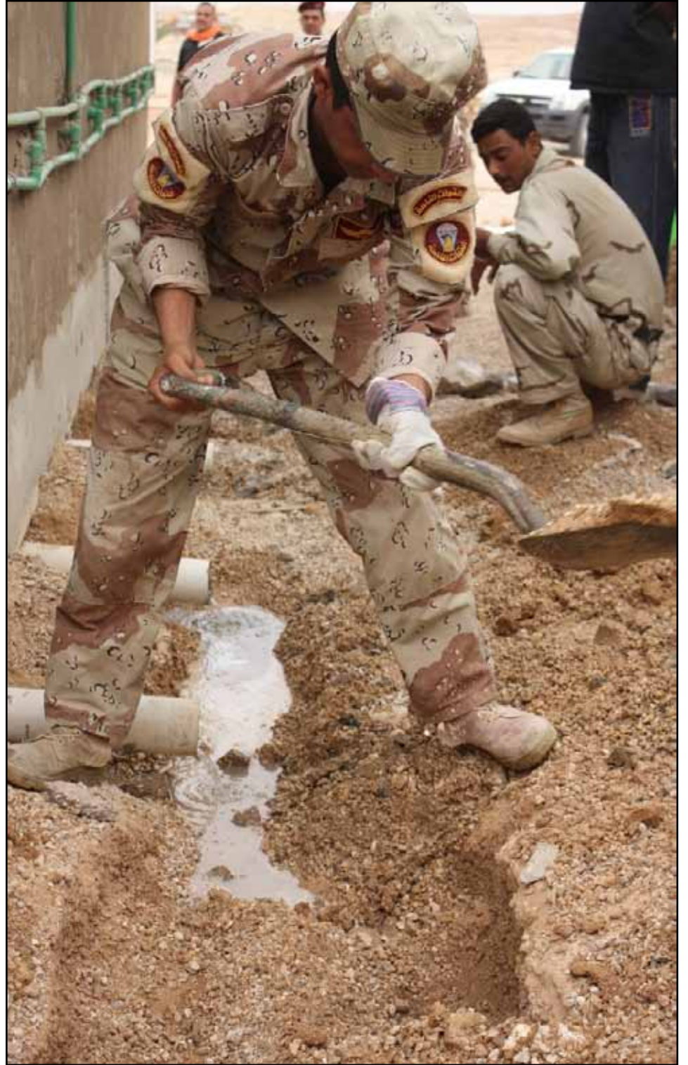
BAGHDAD — A Soldier from the 7th Iraqi Army digs a trench for a new shower drainage pipe at Camp Yassir April 11. Many IA Soldiers have the expertise but lack the confidence to fix basic maintenance issues at the camp.
