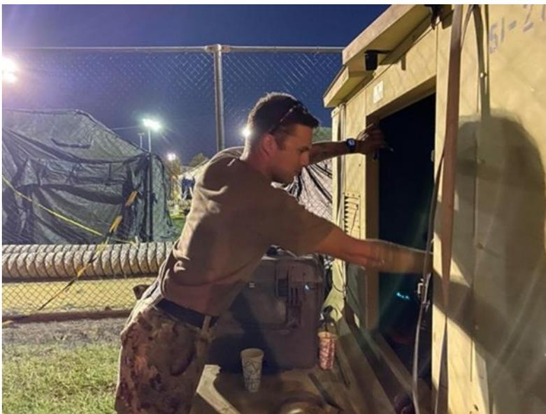
Construction Mechanic 2nd Class Joseph Bergan repairs an environment control unit (ECU) supporting the living facilities constructed for evacuees from Afghanistan at Naval Station (NAVSTA) Rota, Aug. 29, 2021. (U.S. Navy photo by Lt. Chanhan Lee)
