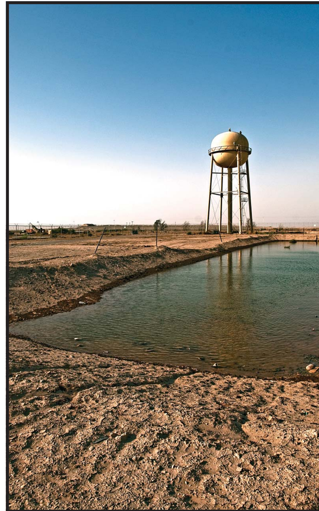
CONTINGENCY OPERATING BASE ADDER FEATURES A WATER TOWER—A RARITY IN SOUTHERN IRAQ—WHICH USES THE POWER OF GRAVITY TO ACCOMPLISH THE MISSION. A PUMP CARRIES WATER UP THE TOWER, AND THEN GRAVITY BRINGS THE WATER DOWN THROUGH THE PIPES AND TO BASE RESIDENTS.
