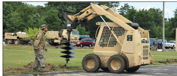
Soldiers with the 409th Vertical Construction Company of Windsor, Colo., work on a troop project June 22 on post.
