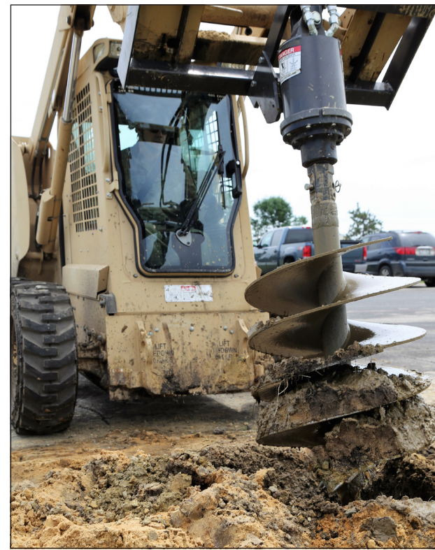
Sgt. 1st Class Donald Ransom, platoon sergeant with the 409th Vertical Construction Company, operates a skid steer with a drilling attachment at the project site.
