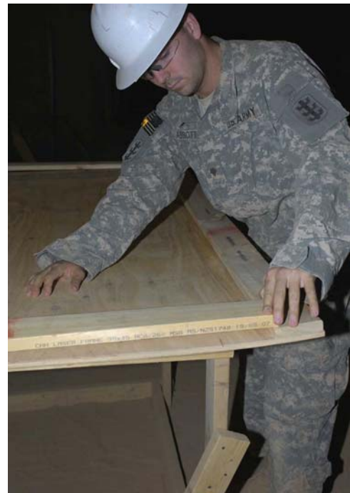
Spc. Corey J. Abbot, of Altus, Okla., a vertical construction specialist with the 643rd Engineer Company makes a door for a housing structure at Combat Outpost India, Mosul, Iraq, July 18. The construction project will house advisory teams to train Iraqi Security Forces.
