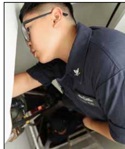
ET3 Ronnica Salas performs maintenance on underwater log equipment.
