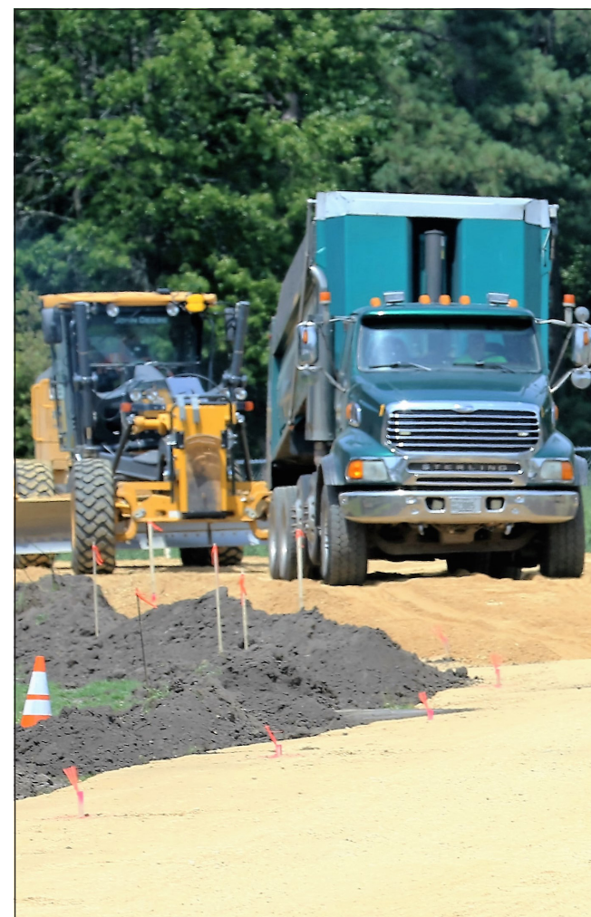
Contractors prepare a driveway and roadway in Constitution Park for paving July 12 at Fort McCoy.
