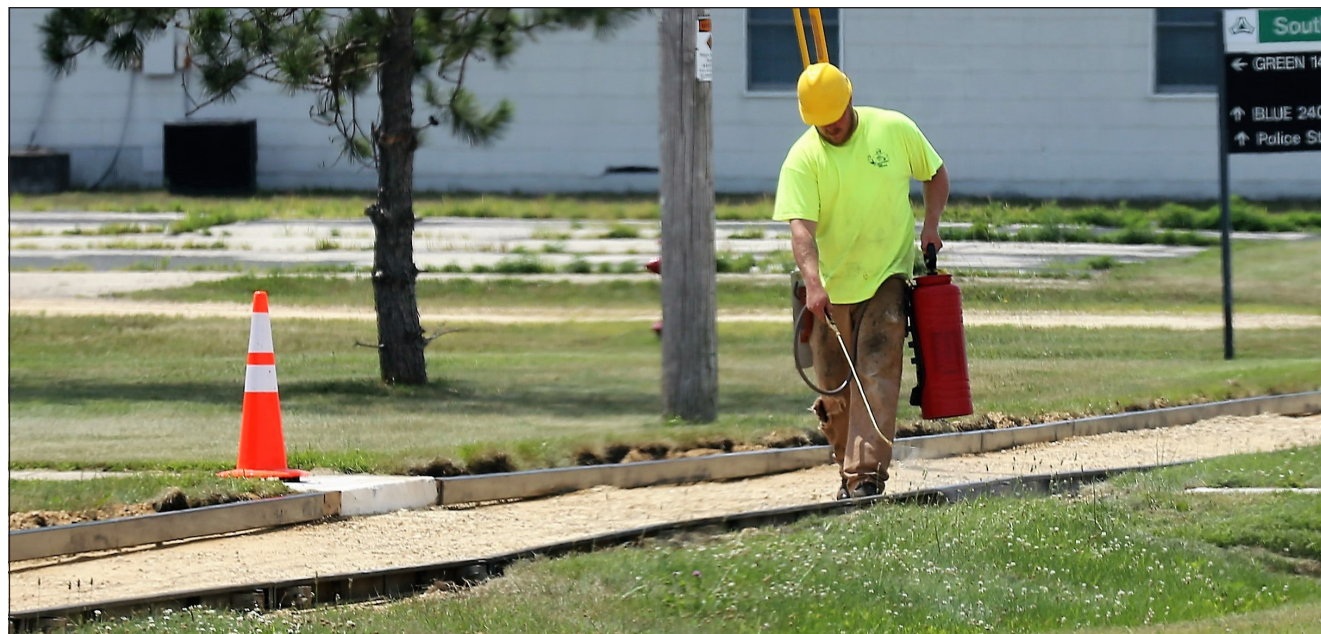
A contractor prepares an area for a new sidewalk to be filled with cement July 12 near the 1100 block at Fort McCoy.
