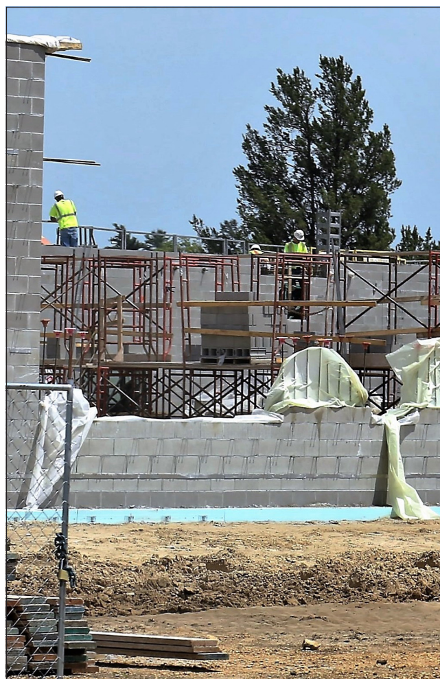
Contractors work on a new $13.5 million, 1,428-person annual training/mobilization dining facility July 12 in the 1800-block at Fort McCoy.
