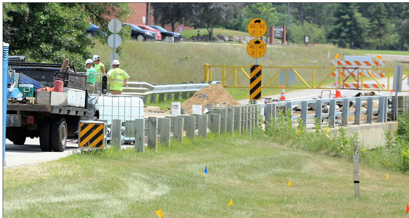
Contractors work on a bridge July 12 near the Wisconsin State Patrol Academy that needed repairs following a 2016 inspection.
