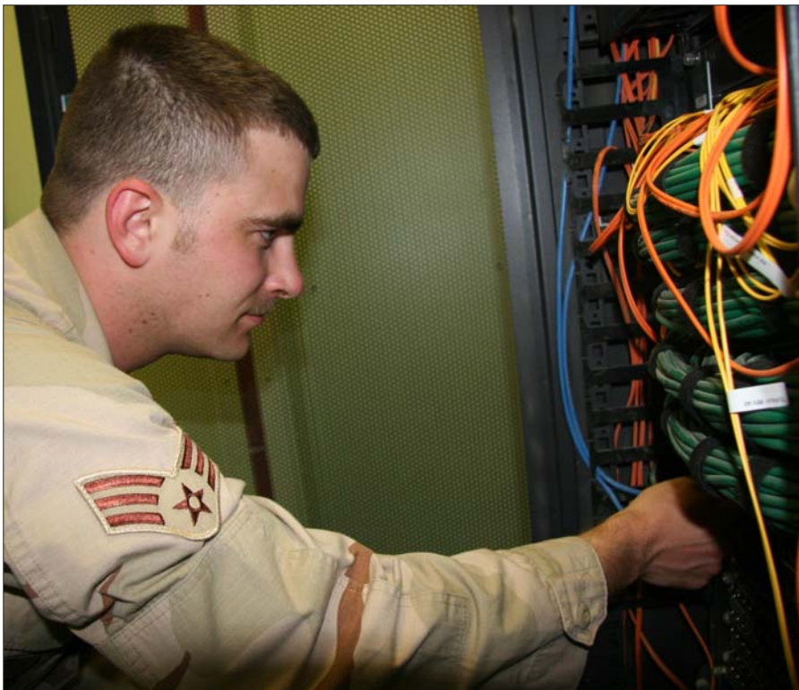
SrA Jason Menningen, 407th ECS computer systems controller, attaches a CAT 5 cable to the network switch.
