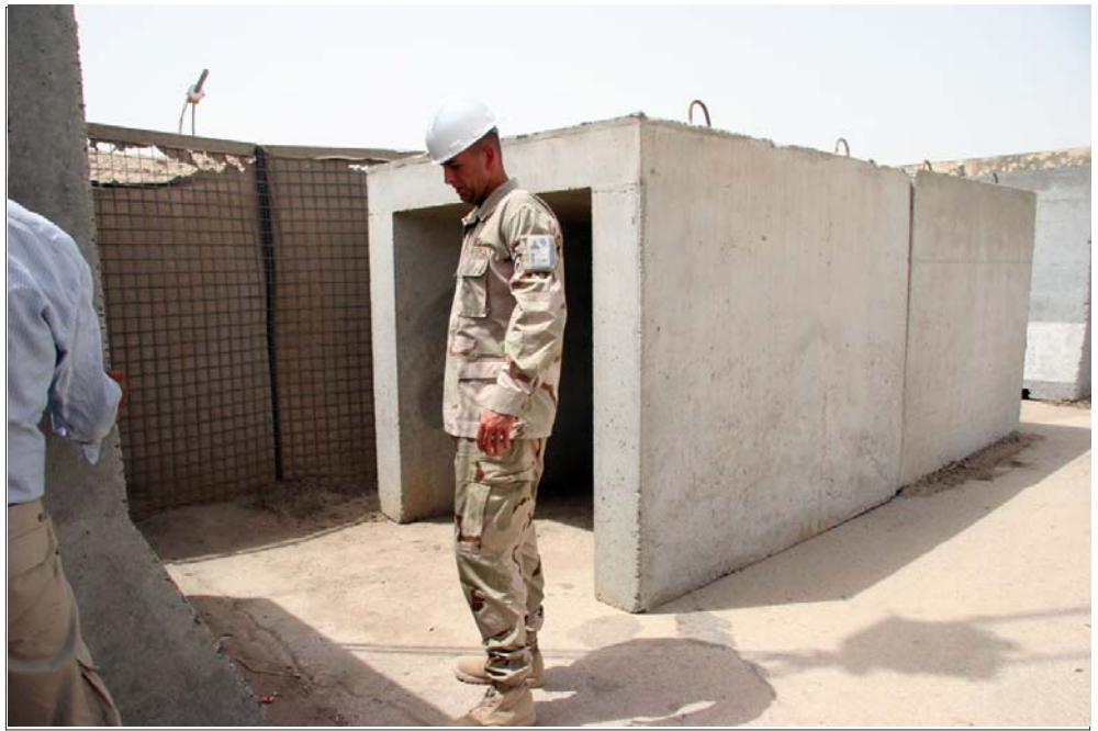
Senior Airman Thomas Ard, 407th ECES, monitors the contractors who are placing a t-wall at one of the entrances to a bunker barrier at the passenger terminal, July 31.
