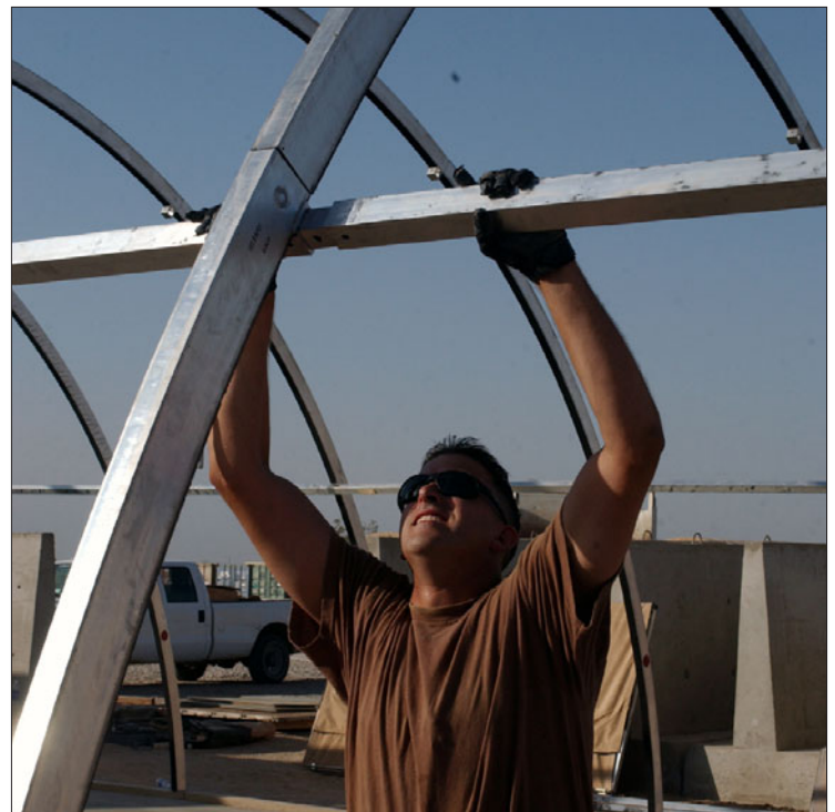
Sergeant Martin pins together the frame of a pre-built shelter. (Photo by Master Sgt. Andrew Gates)
