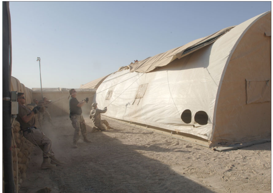
Staff Sgt. Jonathan Martin, Staff Sergeant Sean Winchcombe and the rest of the structures team pull the cover for a California shelter over the skeleton. (Photo by Staff Sgt. Rasheen Douglas)
