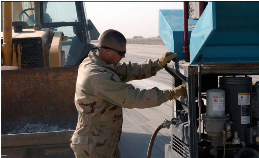
Staff Sgt. Sean Italiane starts the compressor to run the jackhammer to break up runway pavement.
