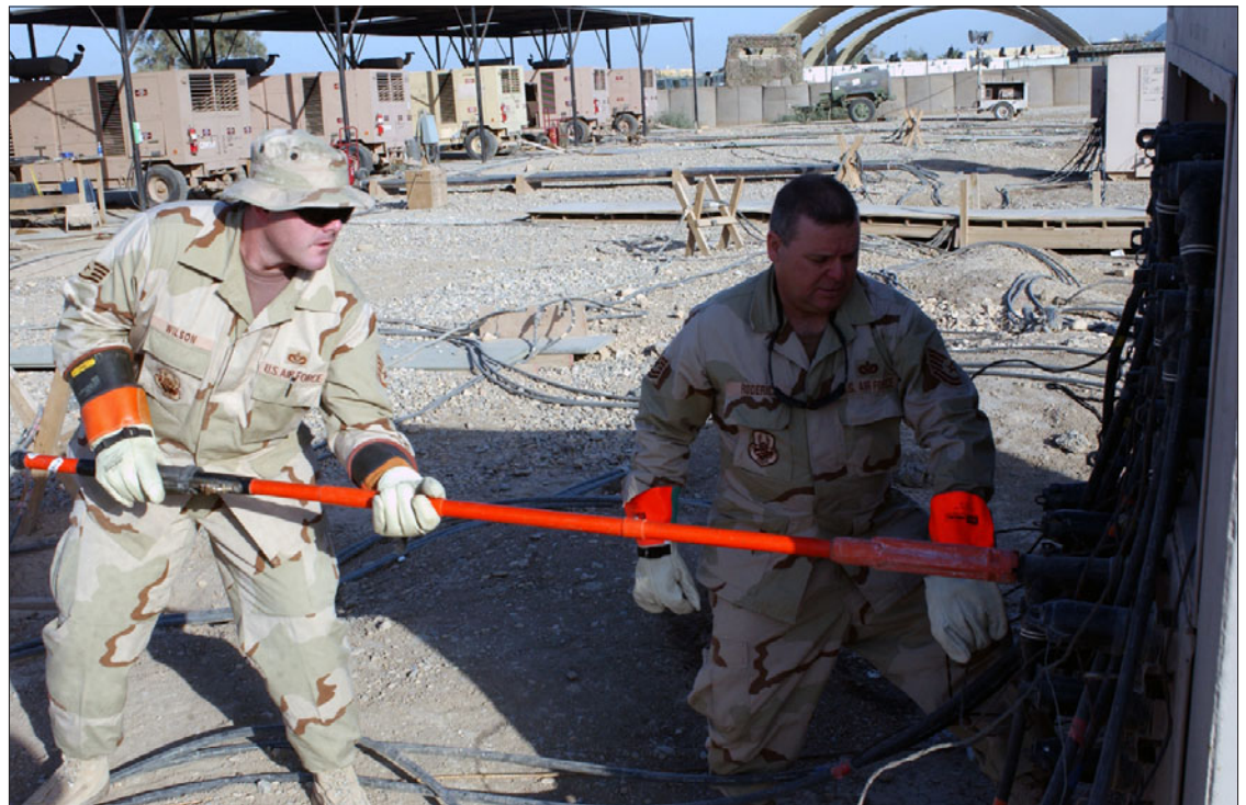
Staff Sgt. James Wilson, left, and Tech. Sgt. James Roderick, 407th Expeditionary Civil Engineer Squadron electricians connect, or “park,” a generator on the primary distribution center. Parking a generator means connecting it to the distribution center before the generator is started. (Photo by Master Sgt. Andrew Gates)
