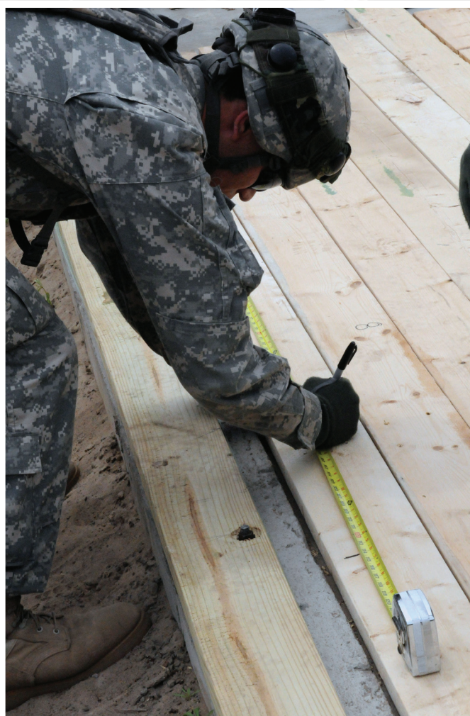
Spc. Ivan Garcia marks a measured piece of lumber prior to cutting it to size for the building project at a Combat Support Training Exercise. The building project will train engineers with a real-world construction of a two-story structure which will be used for future training exercises here.
