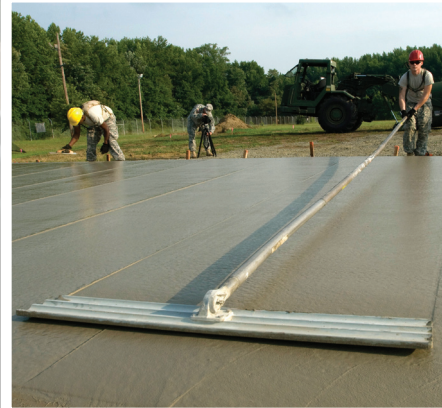
Top) Sgt. Brandon Kidwell, 733rd EN CO, takes a moment to drink some water while working on a 50-man classroom/Kelly building during Castle IRC 2011. Heat index reached well over 110 degrees during most days of the training exercise.
