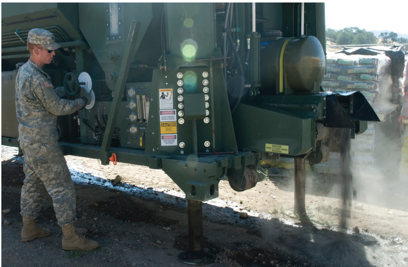
Spc. Kody Misinco, light-wheeled vehicle mechanic, 448th Engineering Detachment, turns the handle on a concrete mixer during Castle Installation Related Construction at Fort Hunter Liggett, Calif., Aug. 3. Misinco is preparing the concrete mixer and doing maintenance to make sure it will be mission capable.
