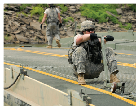
Pvt. Derek Aukes, of the 652nd Engineer Company, located in Hammond, Wis., helps disconnect the bridge bays on the Arkansas River while training during River Assault 2011 at Fort Chaffee, Ark., July 26. (Photo by Spc. Brittney Bradley, 343rd MPAD)
