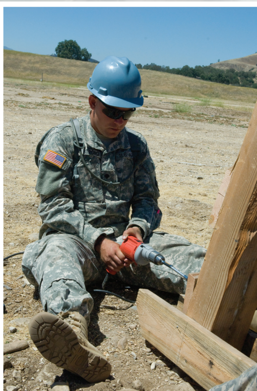
Spc. Trevor D. Strong, 336th Engineering Company, drills a screw into the wood for the base of a guard tower during Castle Installation Related Construction at Fort Hunter Liggett, Calif. Aug. 2.
