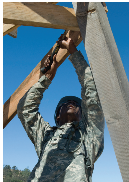
Top) Pvt. Corey Duke, 336th Engineering Company, prepares to nail together two wooden boards during Castle Installation Related Construction at Fort Hunter Liggett, Calif. Aug. 2.
