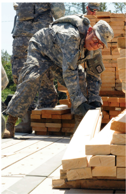
Cpl. Robert Roth with the 284th EN CO prepares to hand lumber down to fellow engineers during a build of materials during Combat Support Training Exercise. Roth lives in Albuquerque, N.M. The build of materials was in preparation to the engineers constructing a two-story structure at the site in the future.
