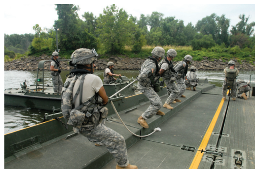
Soldiers of the 652nd Engineer Company, located in Hammond, Wis., remove tension in bridge bays before disconnecting them on the Arkansas River as part of a training event at River Assault 2011 at Fort Chaffee, Ark., July 26. (Photo by Spc. Brittney Bradley, 343rd MPAD)
