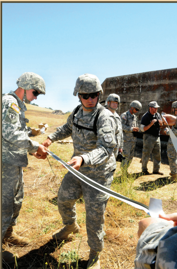
Spc. Zach Batista (right), Headquarters and Headquarter Company, 315th Engineer Battalion, combat engineer from Chino, Calif., adjusts the detonating cord on duct tape to place on the hinges of a door, while Pfc. Travis Davis, 336th Engineer Detachment, electrician, from Enon Valley, Pa. holds the tape tight. The soldiers were at a combat engineer demolition range Aug. 9 at Fort Hunter Liggett, Calif. The engineer Soldiers are attending Castle Installation Related Construction for their annual training. (U.S. Army photo by Sgt. Debralee P. Crankshaw, 363rd PAD)
