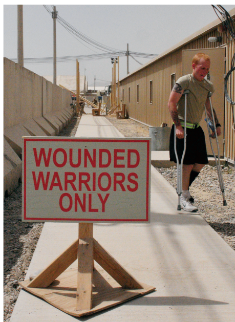
A Soldier walks out of the Wounded Warrior Care Center on Kandahar Airfield. U.S. Navy Seabees (in the background) assigned to Naval Mobile Construction Battalion 1, based out of Gulfport, Miss., work on a walkway deck for the Wounded Warrior care center.
