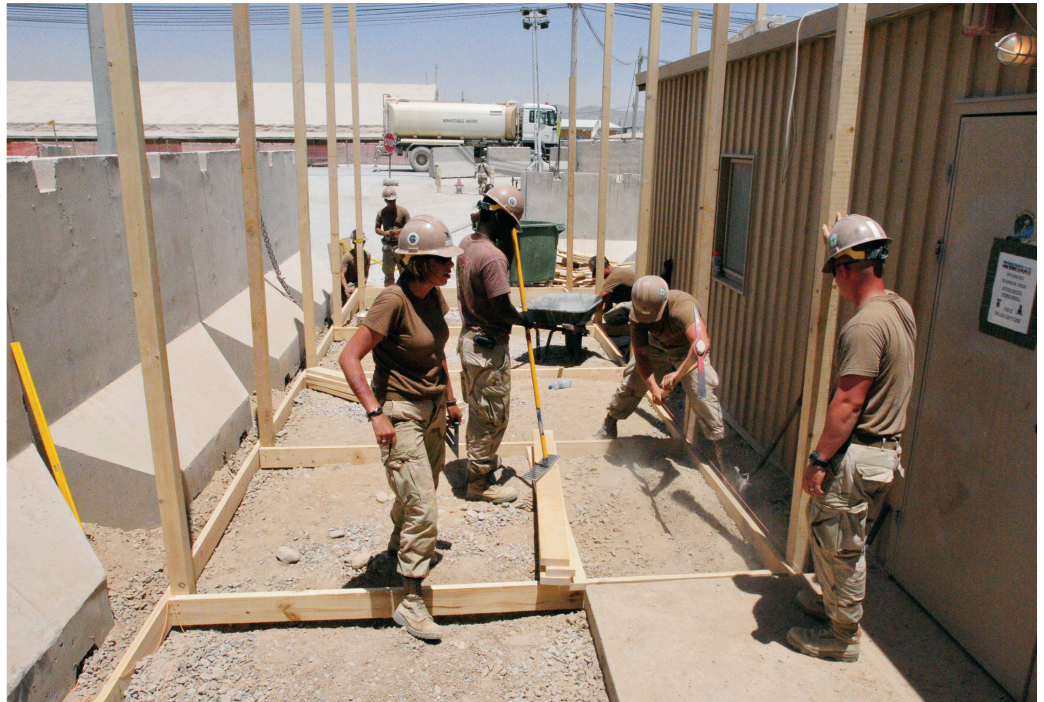
U.S. Navy Seabees assigned to Naval Mobile Construction Battalion 1, based out of Gulfport, Miss., work on what will become a walkway deck for the Wounded Warrior Care Center on Kandahar Airfield. The boardwalk will make it easier for injured service members to get around without having to trip on rocks or uneven ground.
