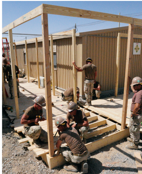
U.S. Navy Seabees assigned to Naval Mobile Construction Battalion 1, based out of Gulfport, Miss., work on what will become a ramp and walkway deck for the Wounded Warrior Care Center on Kandahar Airfield.
