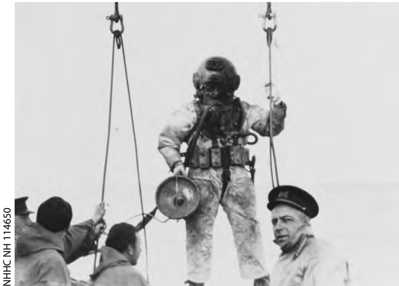
A diver going over the side for salvage activities on USS S-51 (SS-162) with a Westinghouse lamp used for underwater lighting, 1926.
