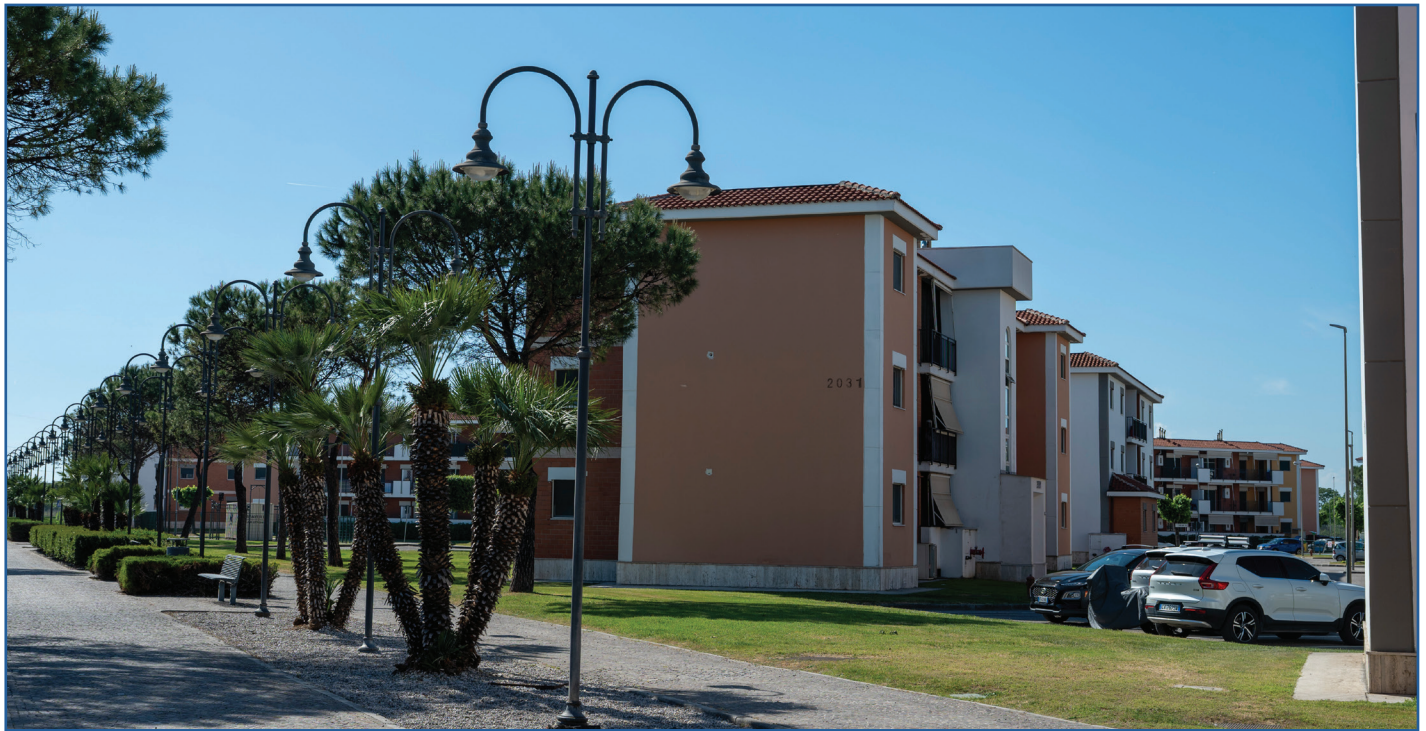
A cross section of family housing units located onboard NSA Naples Support Site.
