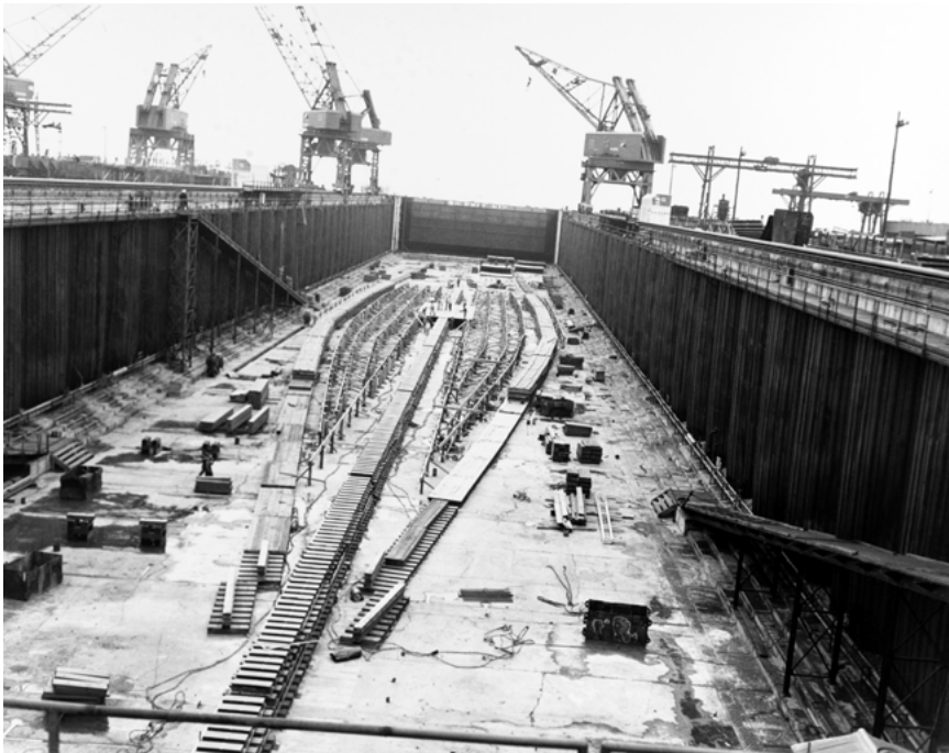
The keel plate of USS United States (CVA-58) being laid in a construction dry dock at the Newport News Shipbuilding and Dry Dock Company shipyard, Newport News, Virginia, 18 April 1949. The carrier was cancelled a few days later, on 23 April. (NARA, 80-G-707176)
