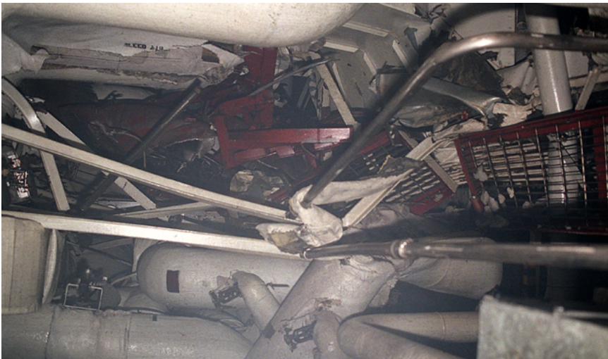
Samuel B. Roberts' main engine room after the mine blast, 1988. (NARA, 6430268)
