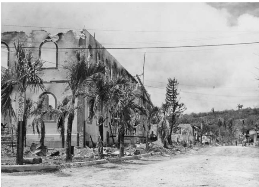
Buildings destroyed by the U.S. Navy's heavy preinvasion bombardment at Agana (present-day Hagåtña), Guam, pictured in July 1944. The largest structure was formerly the best-equipped school on Guam. (NARA, USMC 94045)
