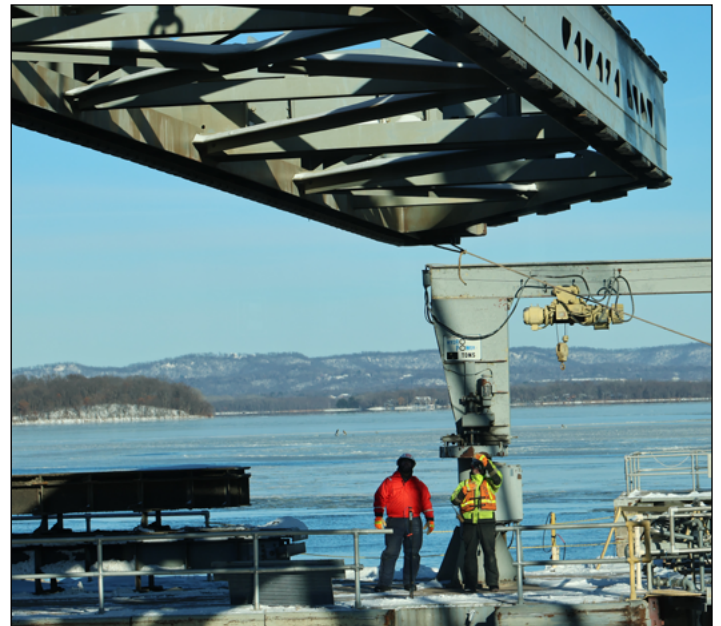
The maintenance and repair crew installs bulkheads at Lock and Dam 7, near La Crescent, Minnesota, to dewater the lock chamber, Dec. 7, 2025. USACE St. Paul District photo by Ren Martin
