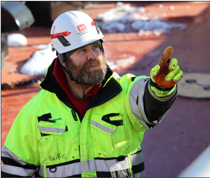
Peter Burke, head operator, works on the bulkhead placement at Lock and Dam 7, near La Crescent, Minnesota, Dec. 7, 2025. USACE St. Paul District photo by Ren Martin
