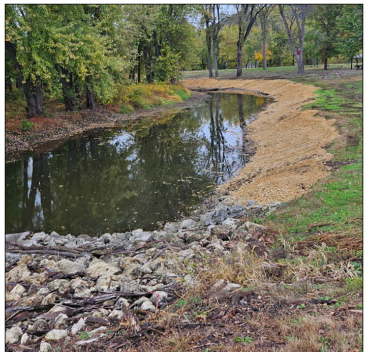
Blackhawk Park shoreline stabilization near DeSoto, Wisconsin, Oct. 22, 2025. USACE St. Paul District courtesy photo
