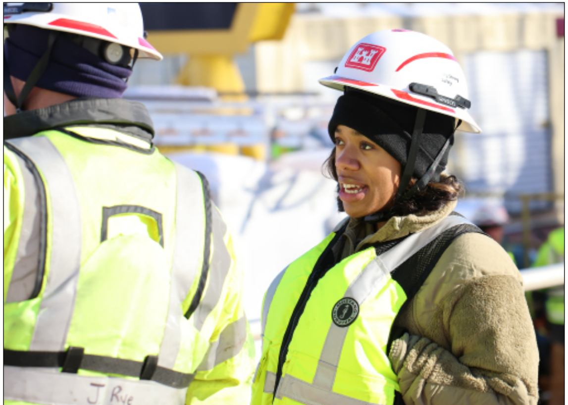
2nd Lt. Shaunna George, industrial hygienist, observes the installation of the bulkheads at Lock and Dam 7, near La Crescent, Minnesota, Dec. 7, 2025. USACE St. Paul District photo by Ren Martin
