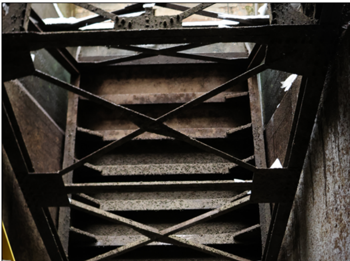
The inside of a Tainter gate, Dec. 18, 2025
