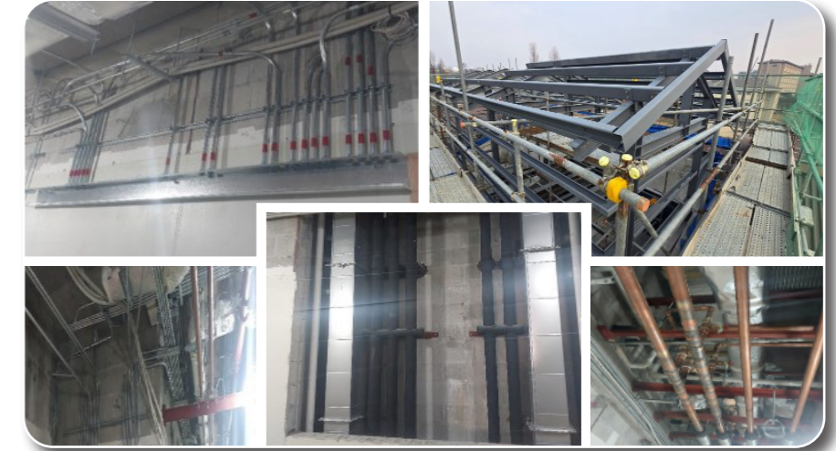
Repair NCO Dormitory B-383, Osan Air Base
