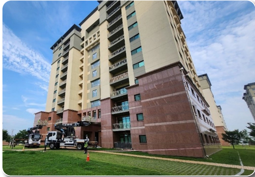
Paint Common Interior Exterior Walls Building 5101, Camp Humphreys
