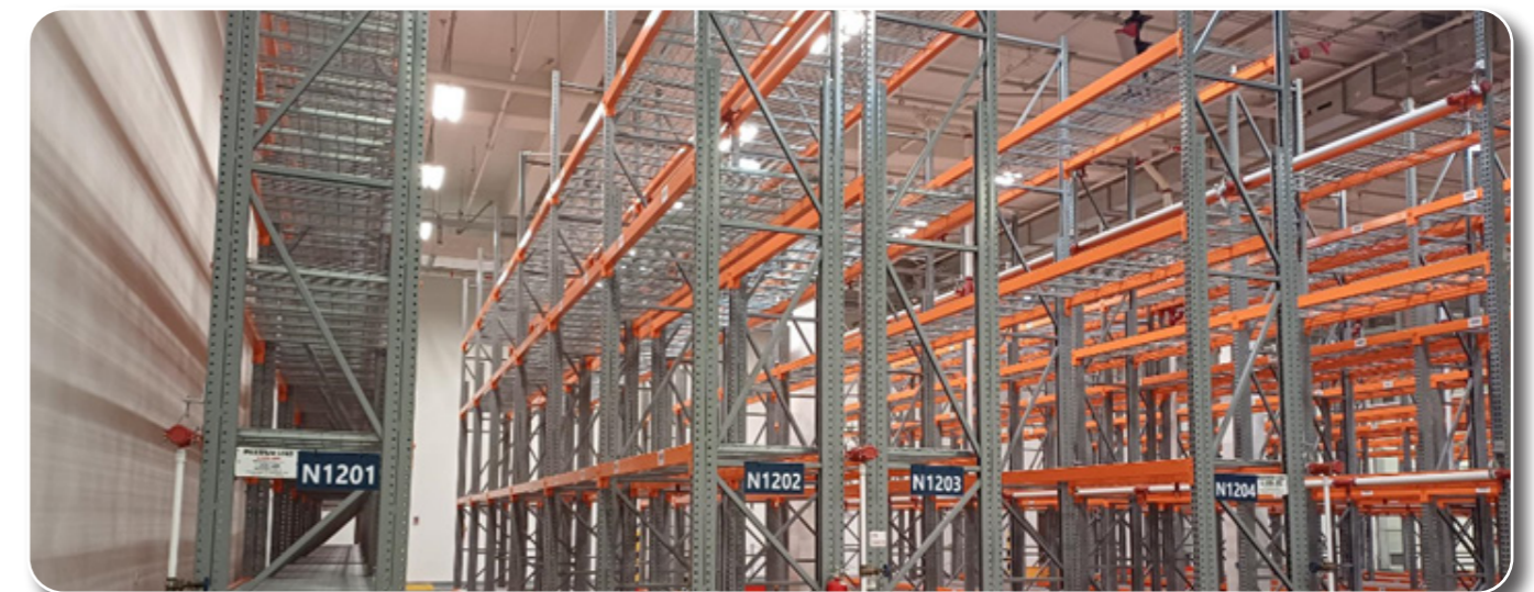
Repair HAZMAT Fire Suppression System at B-586, Camp Carroll
