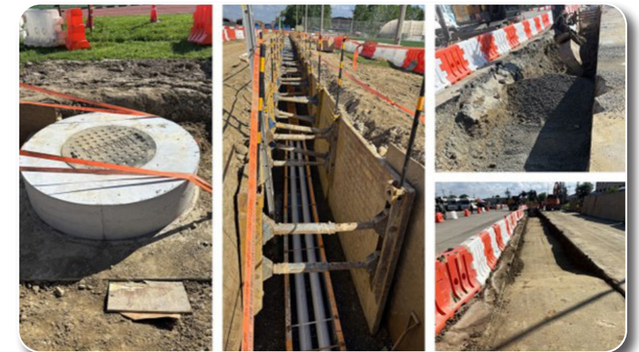
Upgrade Electrical Distribution West Area Phase 3, Osan Air Base
