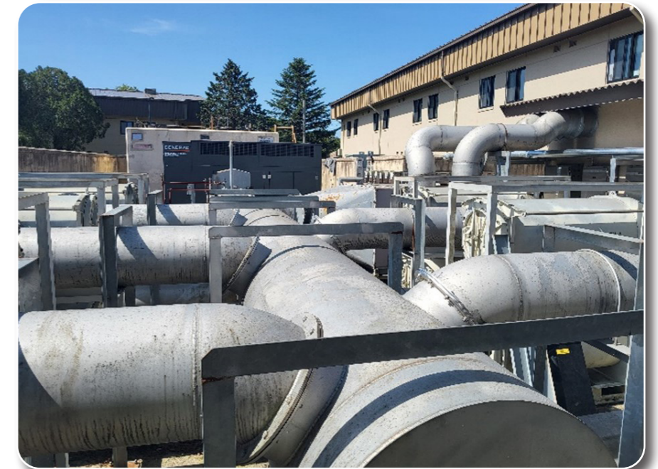
Upgrade Collective Protection System at Dormitories 339 and 1431, Kunsan Air Base
