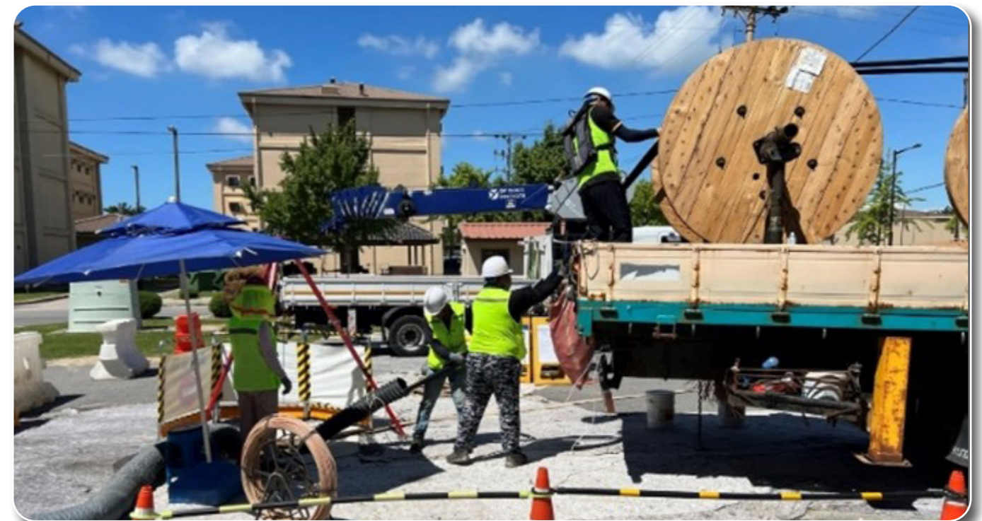
Upgrade Electrical Distribution System, Kunsan Air Base
