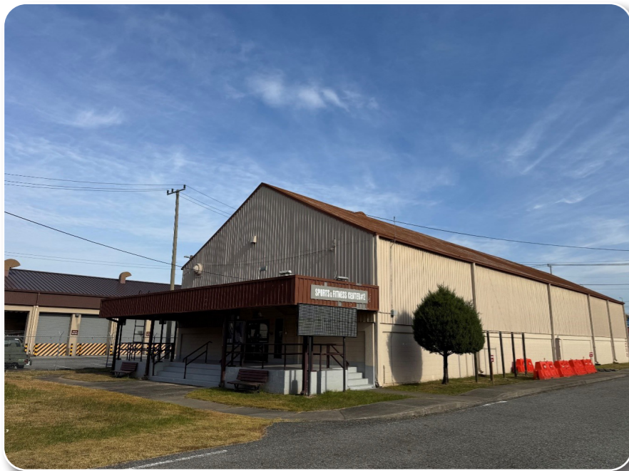
Repair Gymnasium, B-2204, Suwon Air Base
