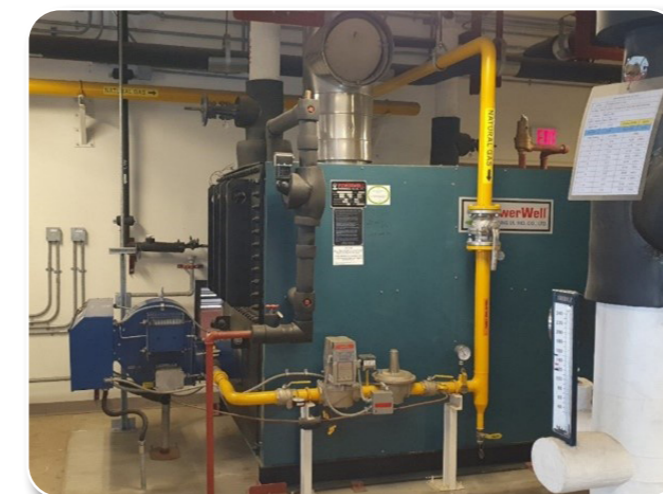
Repair boilers, P-738, P-739 and P-740, Camp Humphreys
