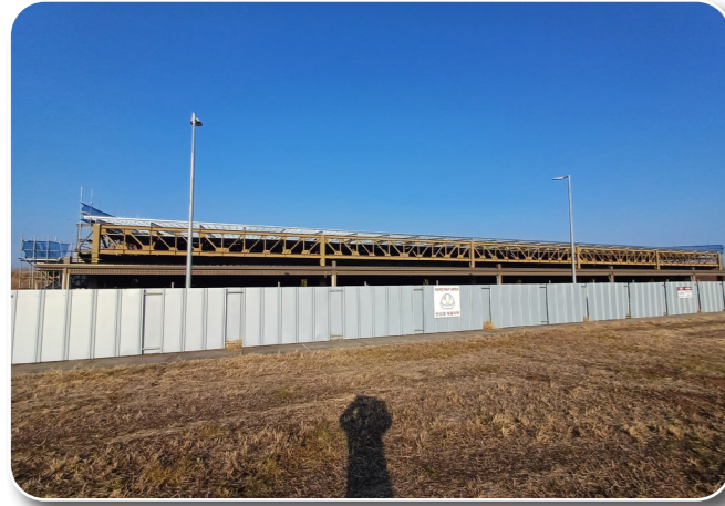
Repair Firing Range Facility P-8350, Camp Humphreys
