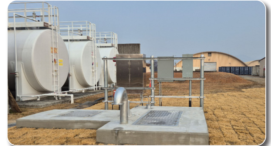
Connect Sewer Lines to ROKAF System, Gimhae Air Base
