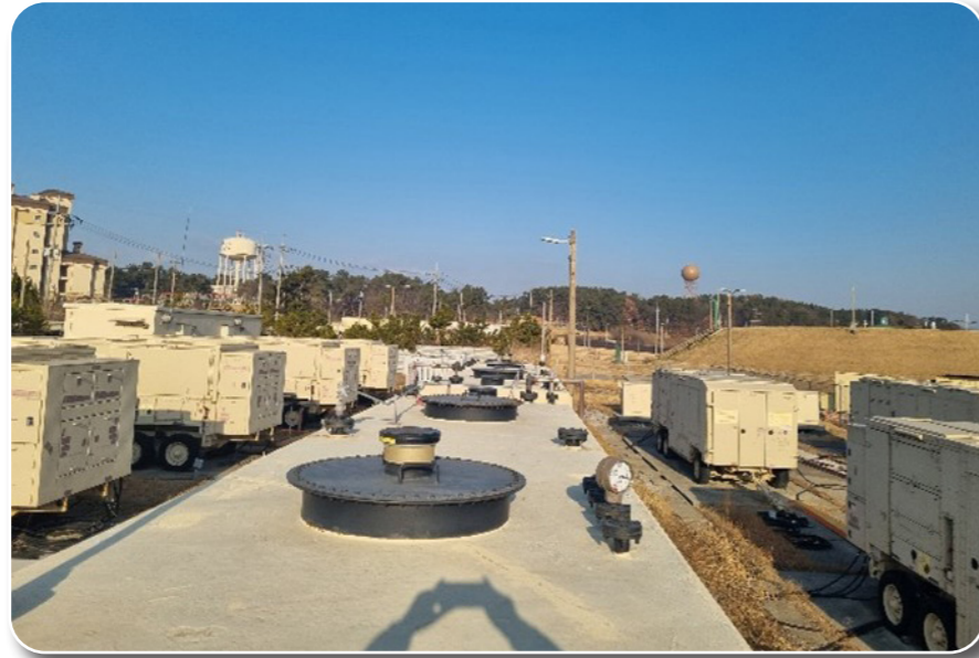
Construct Backup Generator Plants, Kunsan Air Base
