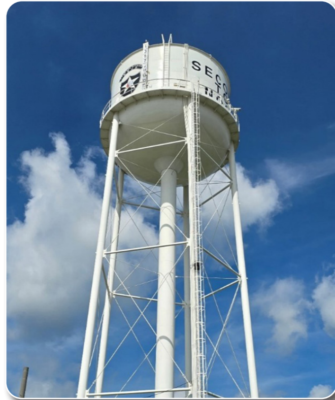
Repair & Coating for Four Elevated Water Towers, Camp Humphreys
