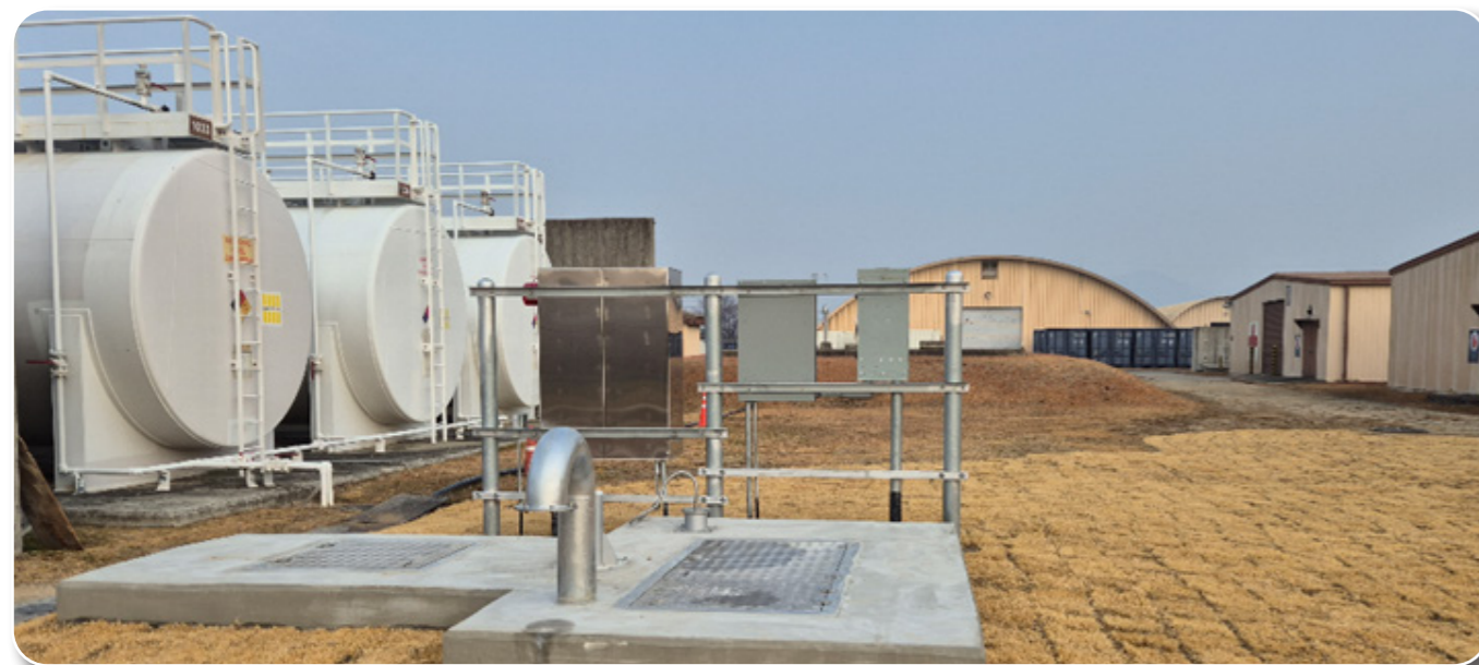
Connect Sewer Lines to ROKAF System, Gimhae Air Base
