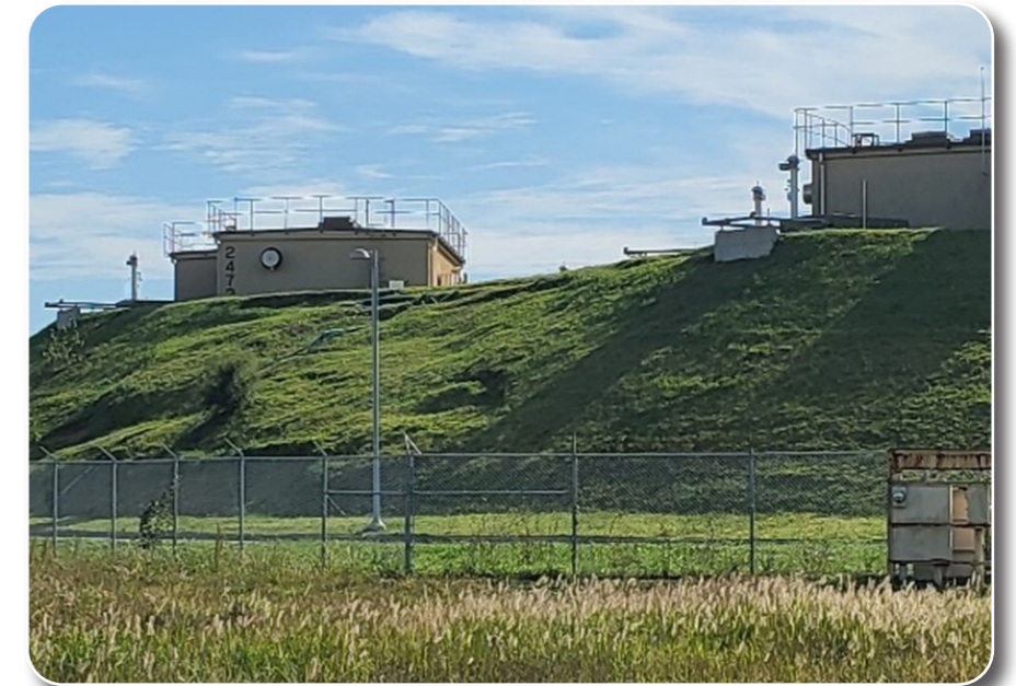
Repair Erosion at Panton Tanks, Kunsan Air Base
