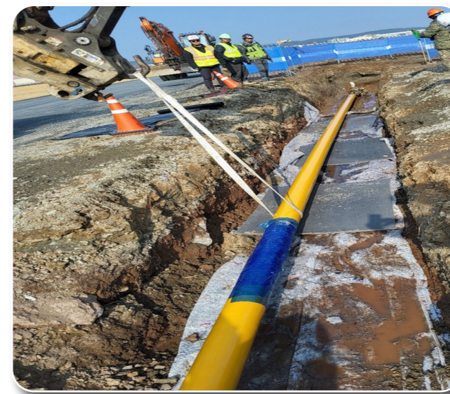
POL Transfer Line Replacement at Kunsan Air Base
