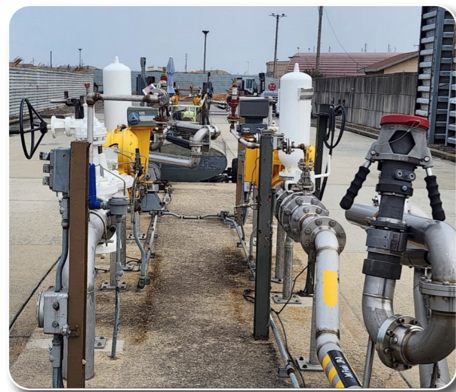
Facility Repair at Kunsan Air Base
