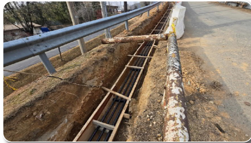
Upgrade Electrical System, Phase II, Camp Carroll
