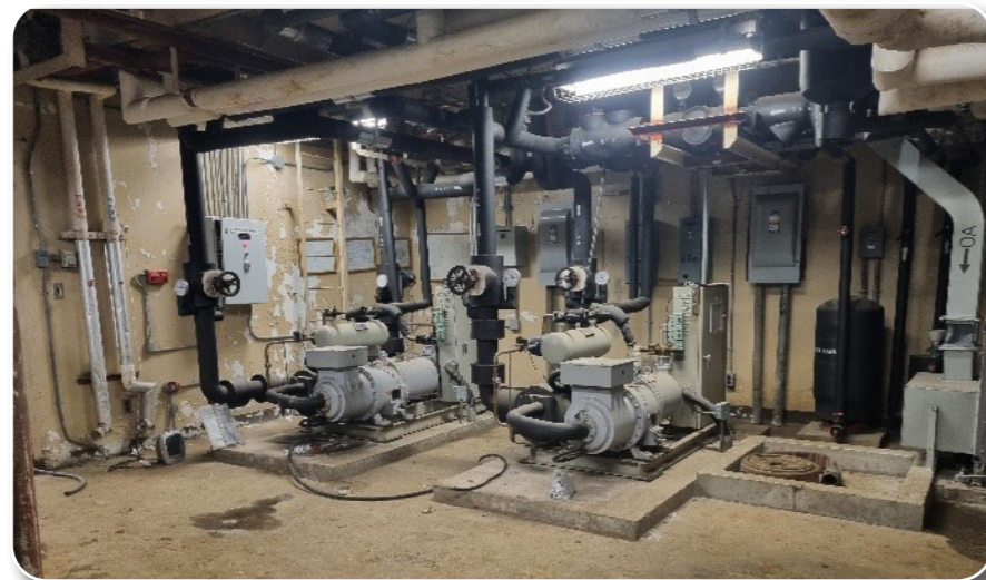
Renovate Aircraft Maintenance Unit (AMU), B-915, Kunsan Air Base
