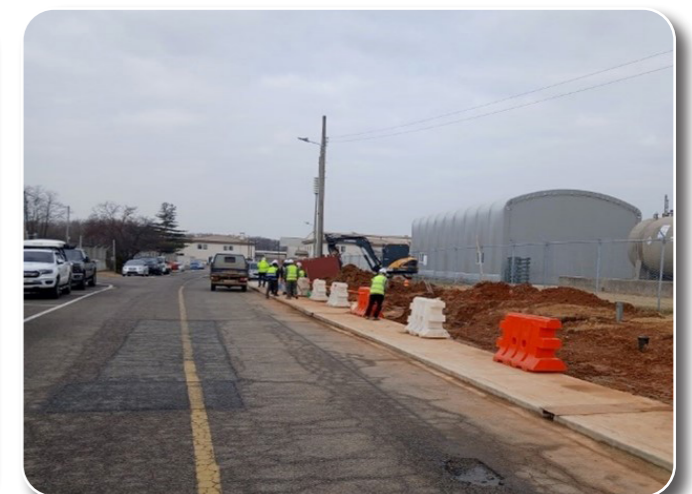
Excavation and Pipe Installation, Camp Humphreys
