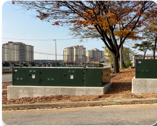
Replace Existing Electrical Pad-Mounted Junctions with Pad-Mounted Switches, Camp Humphreys
