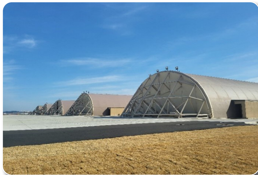
Construct 3rd Generation Hardened Aircraft Shelters, Phase 4, 5, 6, Kunsan Air Base
