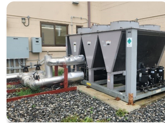
Repair Chillers, P-6322, P-6323 and P-1201, Camp Humphreys
