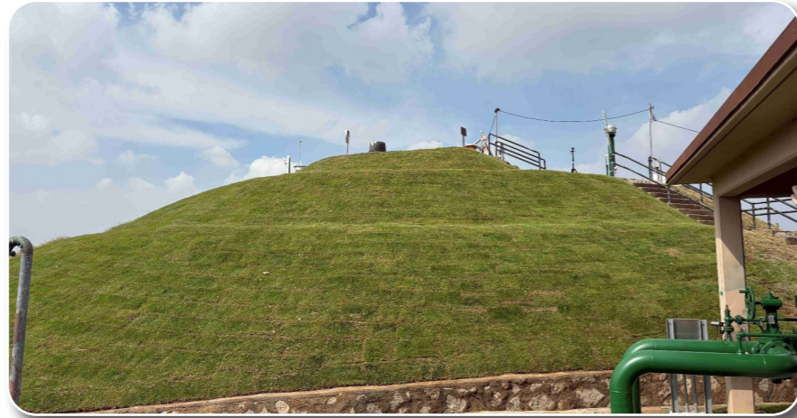
Repair POL Tank 2662, Suwon Air Base
