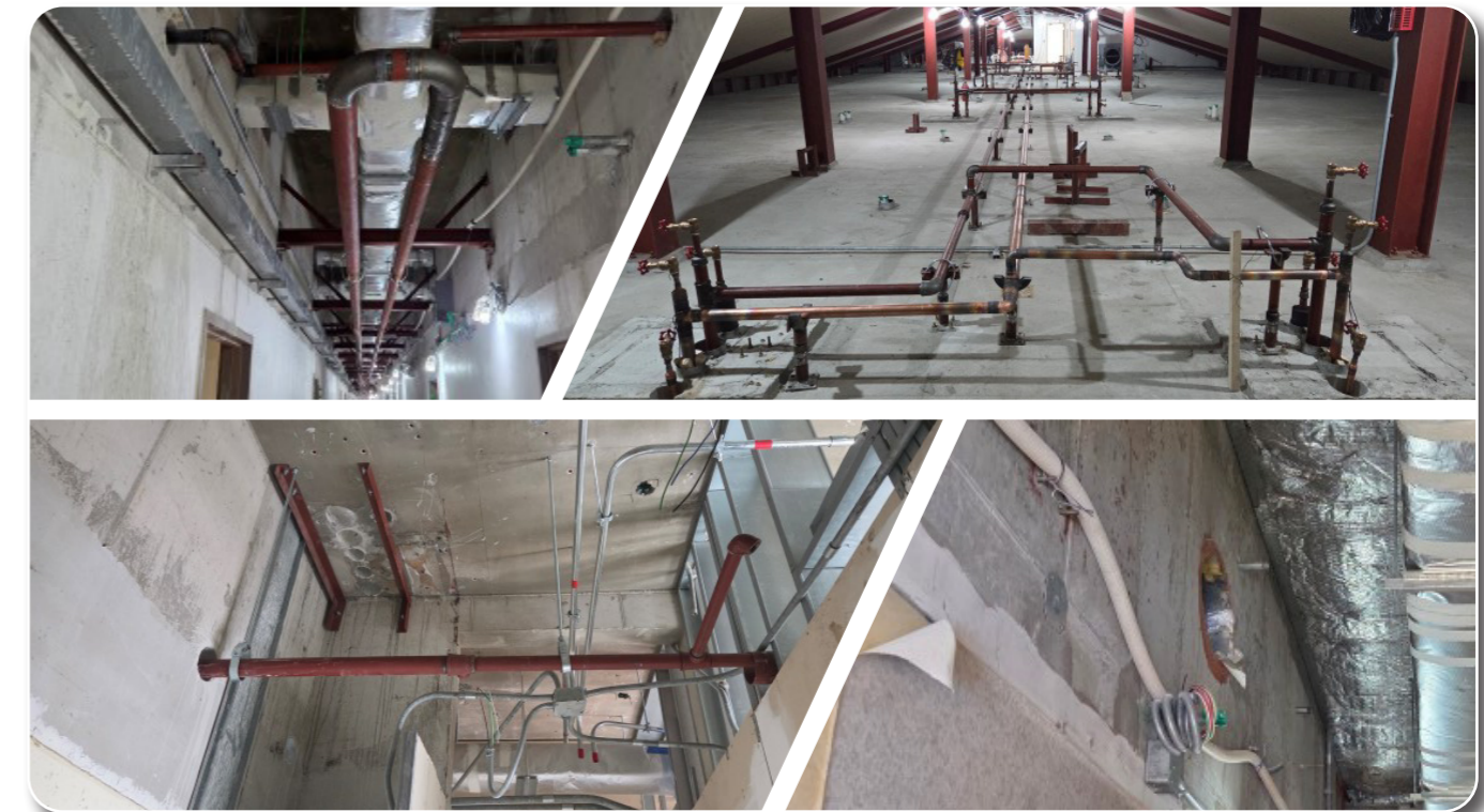
Repair Airmen Dormitory B-1458, Osan Air Base
