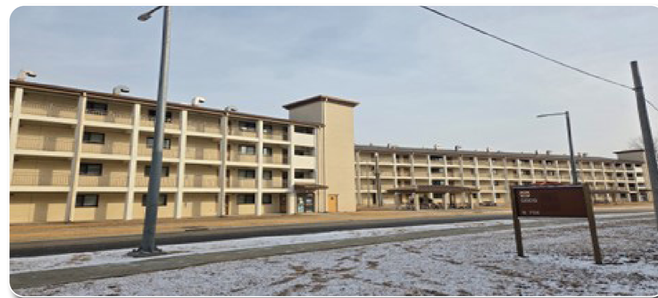
Repair Plumbing System, 3 Barracks, P-753, 754, & 755, Camp Humphreys
