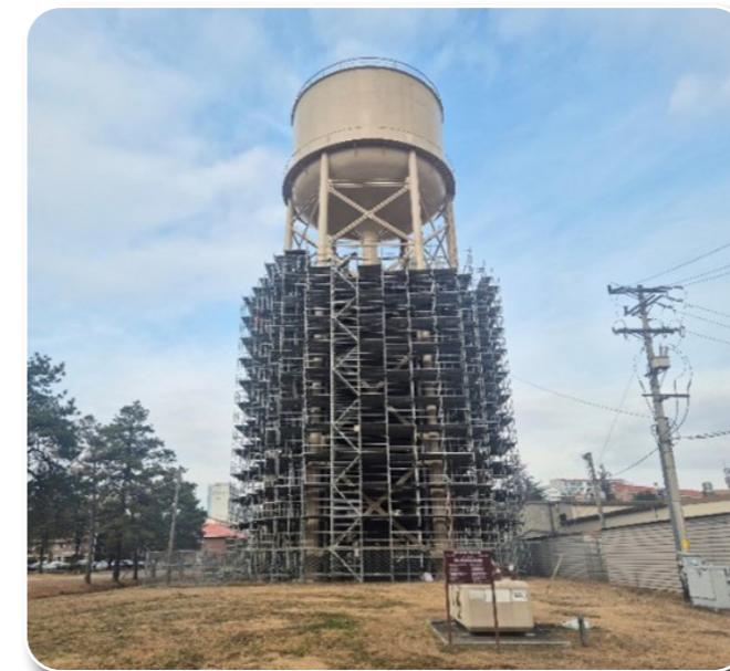
Repair Elevated Steel Water Storage Tank, Gwangju Air Base
