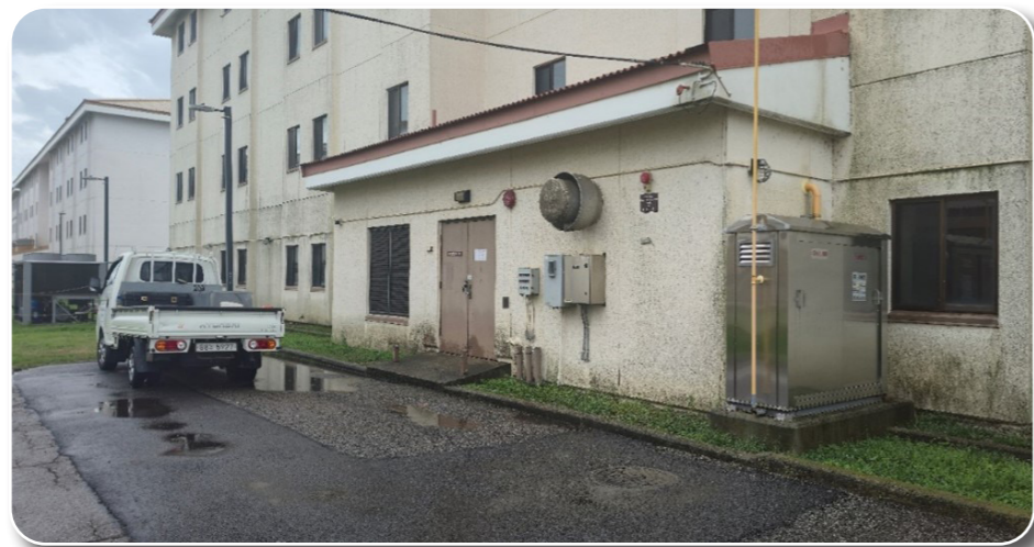
Replace HVAC Equipment and Piping P-1057, Camp Humphreys
