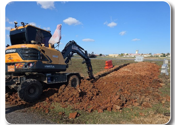
Replace Asbestos Water Lines in Legacy Area, Camp Humphreys
