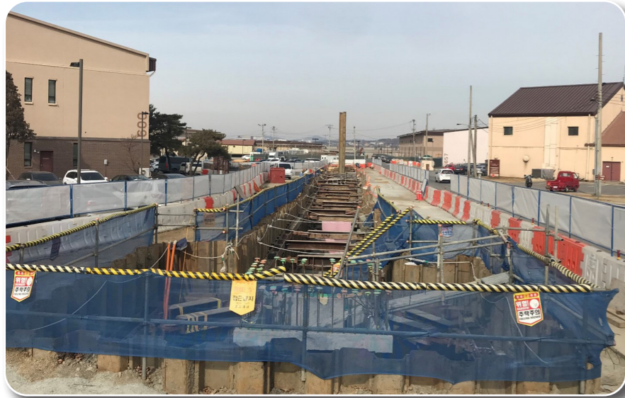
Repair Sewer Lift Station B-659, B-823, B-1706, B-1356, Osan Air Base
