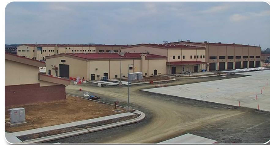
Vehicle Maintenance Facility, Camp Humphreys
