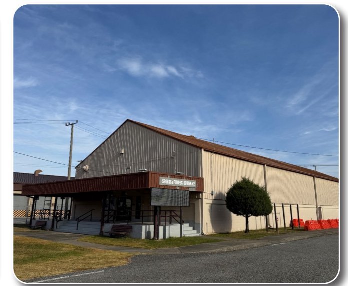
Gymnasium Repair at Suwon Air Base
