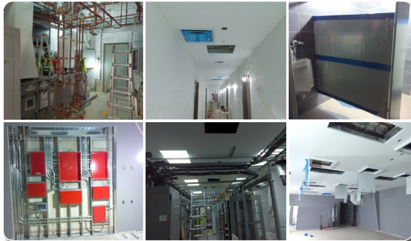
Repair Telecommunications Facility B-2005, Suwon Air Base
