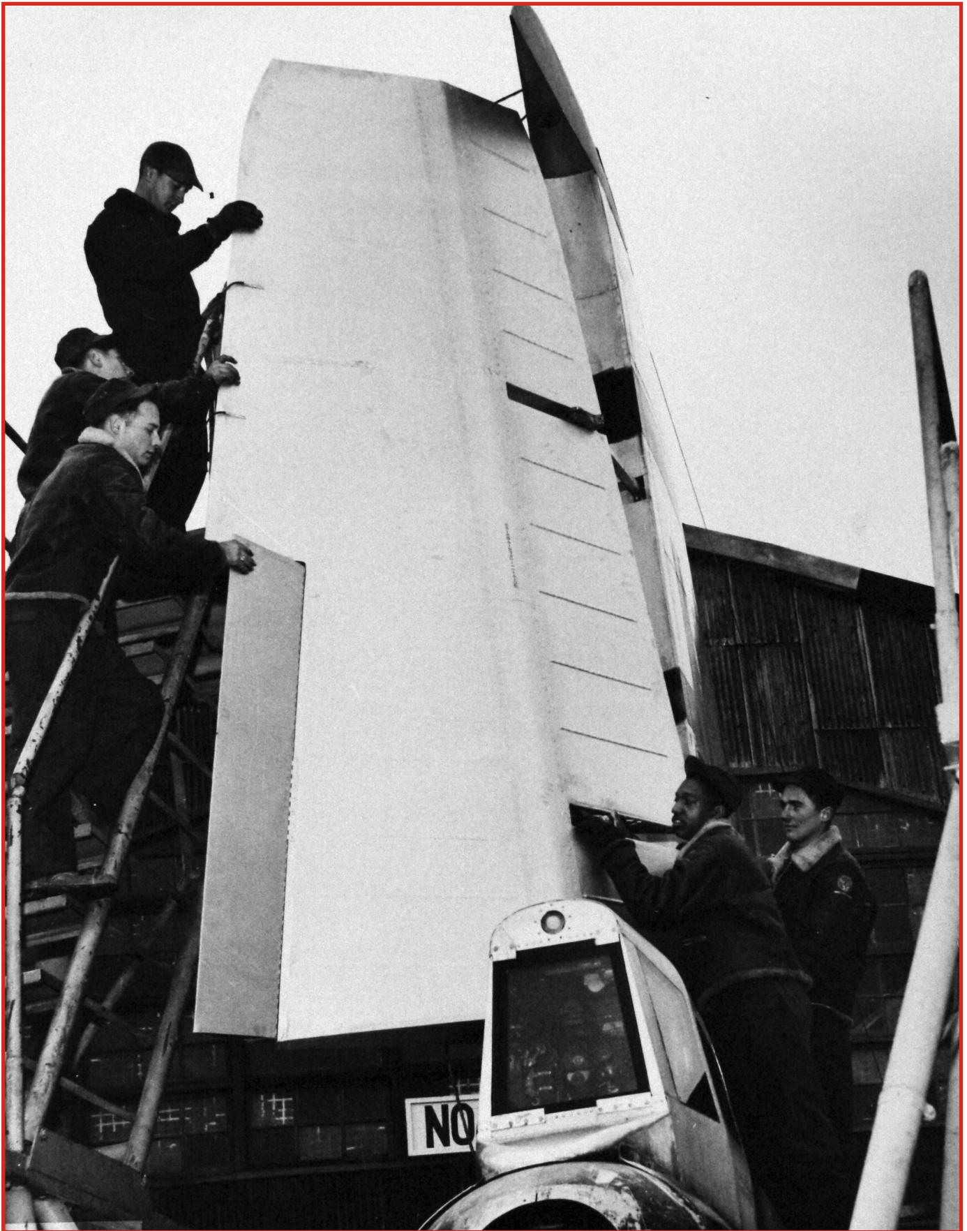
Above: Ground crewman at a U.S. Far East Air Forces B-29 base carefully replace a rudder of a Superfortress. Soon it will fly again to blast the important Communist held sectors of Korea, helping to stave off continued Red drives to push UN forces from the Korean peninsula. January 1951
