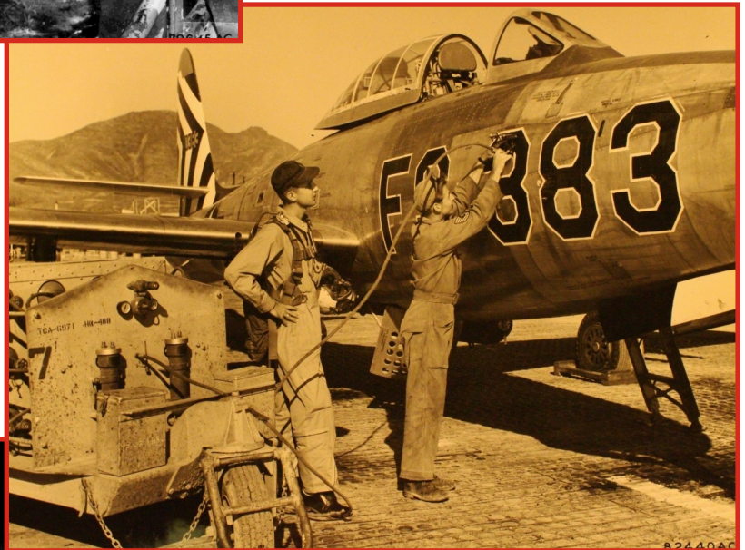
Middle: To assure a steady supply of oxygen for the Far East Air Forces Warcraft, the 6405th Air Support Wing, a Far East Air Logistics Force unit in Korea started producing its own bottled oxygen. Here, 1st Lt. William J. Heath, (left) Cincinnati, Ohio, a U.S. Air Force F-84 "Thunderjet" pilot of the 49th Fighter Bomber Wing, watches his crew chief, T/Sgt. Harold E. Sears of Thomaston, Conn., fill his oxygen tanks. October 1952.
