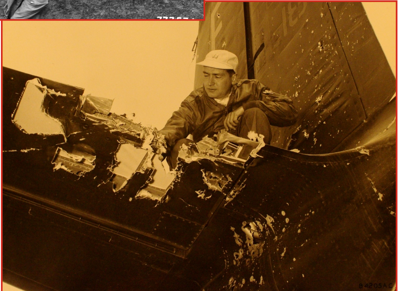
Below: Capt. Alexander M. Lyon, Media, Pa., pilot of the U.S. Air Force 3rd Bomb Wing examines, somewhat unbelievably, his flak-riddled B-26 light bomber, after a safe landing at his base in Korea, when heavy ground fire ripped into the aircraft's tail section. The B-26 was on a night-train-busting mission south of Kyomipo, northeast of Cinnampo in North Korea. Capt. Lyon mounts the riddled tail section for closer inspection of the damage. Two rudder cables were snapped and the elevator section severely damaged by the Red guns. The score for the night: one locomotive damaged and two boxcars destroyed. April 1953.
