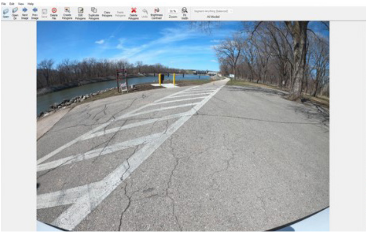
Top: Screenshots of the artificial intelligence program identifying pavement deficiencies from a survey of pavement at a project site.
