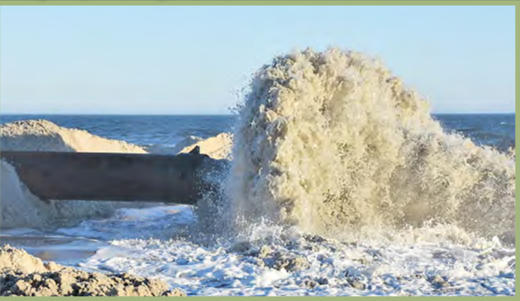
Sand being pumped through pipelines onto Gilgo Beach, one of several beaches receiving sand replenishment with the Fire Island Inlet to Montauk Point, New York, Coastal Storm Risk Management Project. (USACE)
