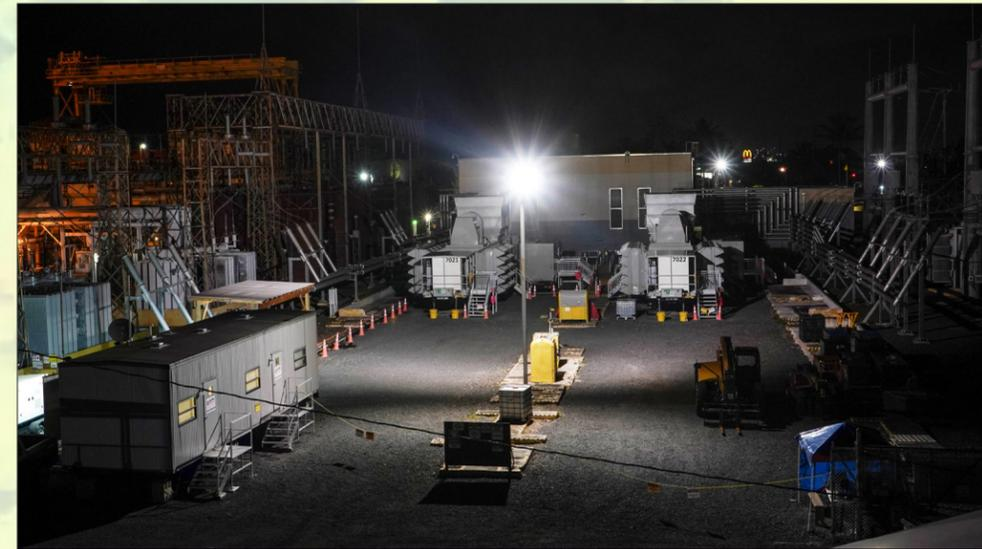
The two generators installed at the Palo Seco Power Plant provided a combined 50 megawatts of power from Oct. 29, 2017, through March 8, 2019.
