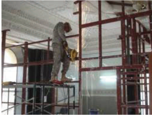
Staff Sgt. Ian Jones, carpenter, Company B, 46th Engineer Combat Battalion (Heavy), a native of Newport, N.Y., uses the rescue saw to cut through steel framing during demolition operations at the Baghdad Operations Command Advisory Team building, January 15.
