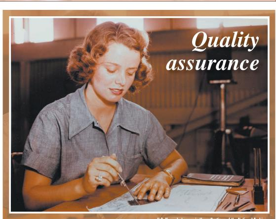
U.S. Navy photo, now in the collections of the National Archives. Aviation Metalsmith 2nd Class Elizabeth Holbrook, USNR (W) checks a finished metal bracket against its blueprint, in a huge assembly and repair building at a naval air station in the Hawaiian Islands,
