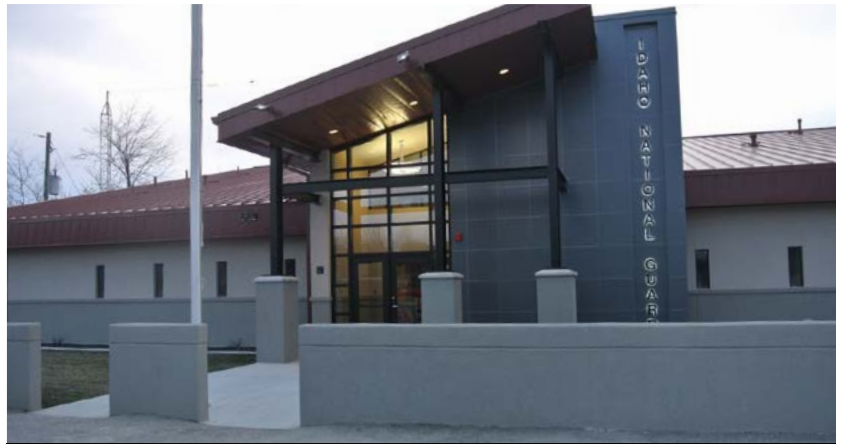
The Emmett Readiness Center was renovated in 2015.
