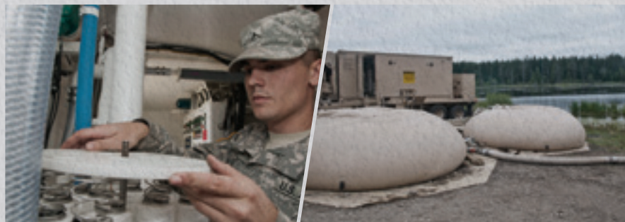
FAR LEFT: Army Pvt. Trevor Swart, with the 651st Quartermaster Company out of Casper, checks the cartridge filters in the 3,000 gallon-per-minute reverse osmosis water purification unit for daily basic preventative maintenance care at Fort Lewis, Wash. (Photo by Sgt. Marco Gutierrez)
