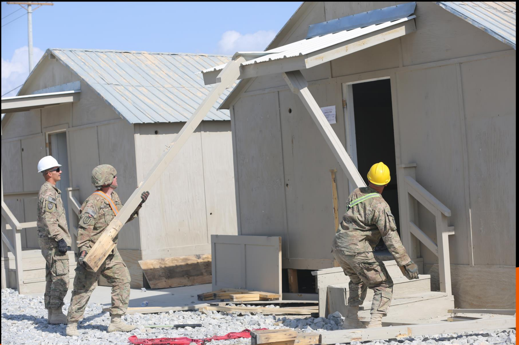
U.S. Army Specialist Ryan Stupp, Jacob Hunn, and Cory Ebel of 304th Engineer Company Vertical and 961st Engineer Company Horizontal tear down buildings on Bagram Air Field, Afghanistan, Oct. 8, 2014. All non-enduring structures are being torn down to reduce sustainment costs and to increase force protection. (U.S. Army photo by Spc. Jamill Ford/Released)
