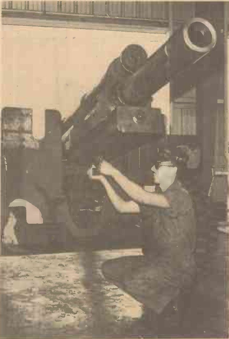
A-OK — Sergeant Ismael Hernandez inspects a 105mm howitzer after reassembly. Three repairmen are capable of disassembling, inspecting, and reassembling the gun in three days.
