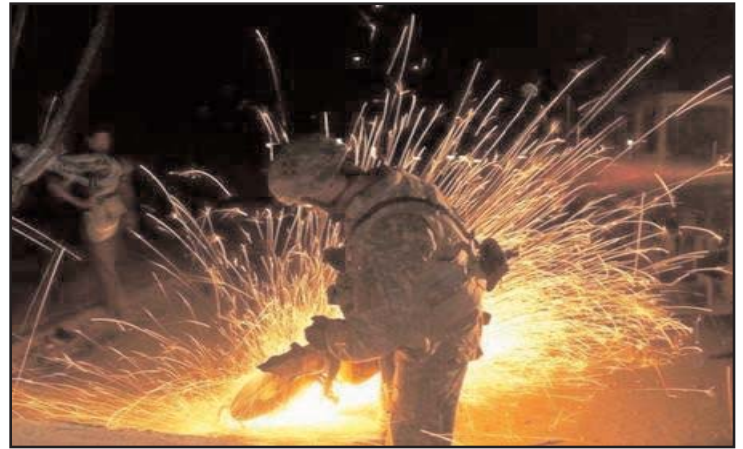
SPC Timothy Adams constructs a Jersey barrier cordon in a dangerous section of East Baghdad by cutting off the rings on the barriers to prevent them from being moved by the local populace.
