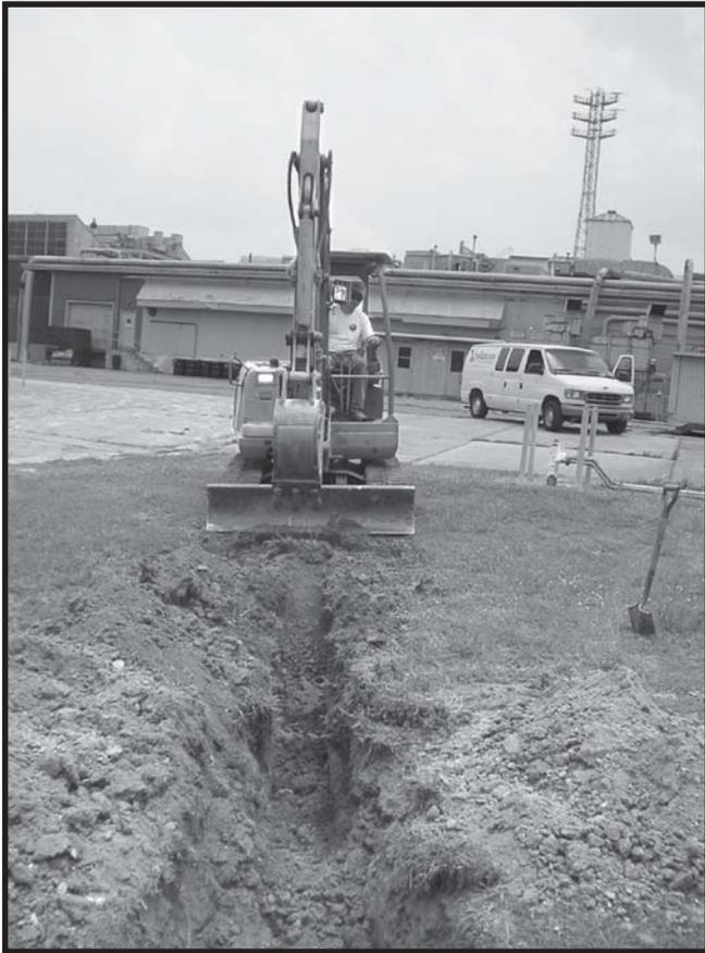
A Solutions-IES employee excavates a trench for the installation of a custom-engineered, below-grade EOS recirculation system.
