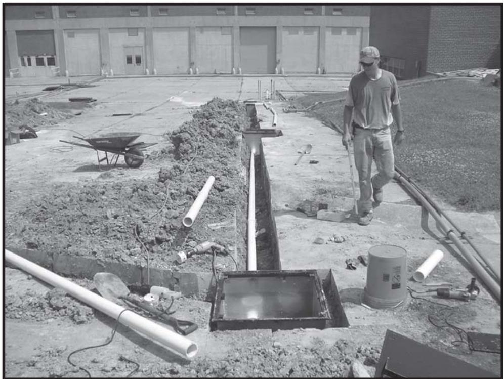
**A Solutions-IES field services manager inspects the installation of EOS injection well vaults. The wells are tied together with double-walled PVC pipes, allowing injections and extractions in alternate wells.**
