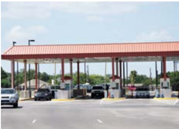
JOINT BASE SAN ANTONIO GATE HOURS
