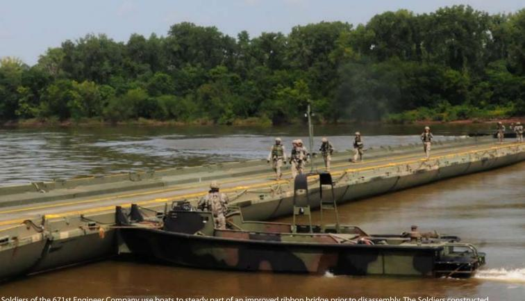
Soldiers of the 671st Engineer Company use boats to steady part of an improved ribbon bridge prior to disassembly. The Soldiers constructed the bridge across the Arkansas River with the 341st Engineer Company during Operation "River Assault" 2010. River Assault is an engineer training exercise conducted annually by the 412th and 416th Theater Engineer Commands.
