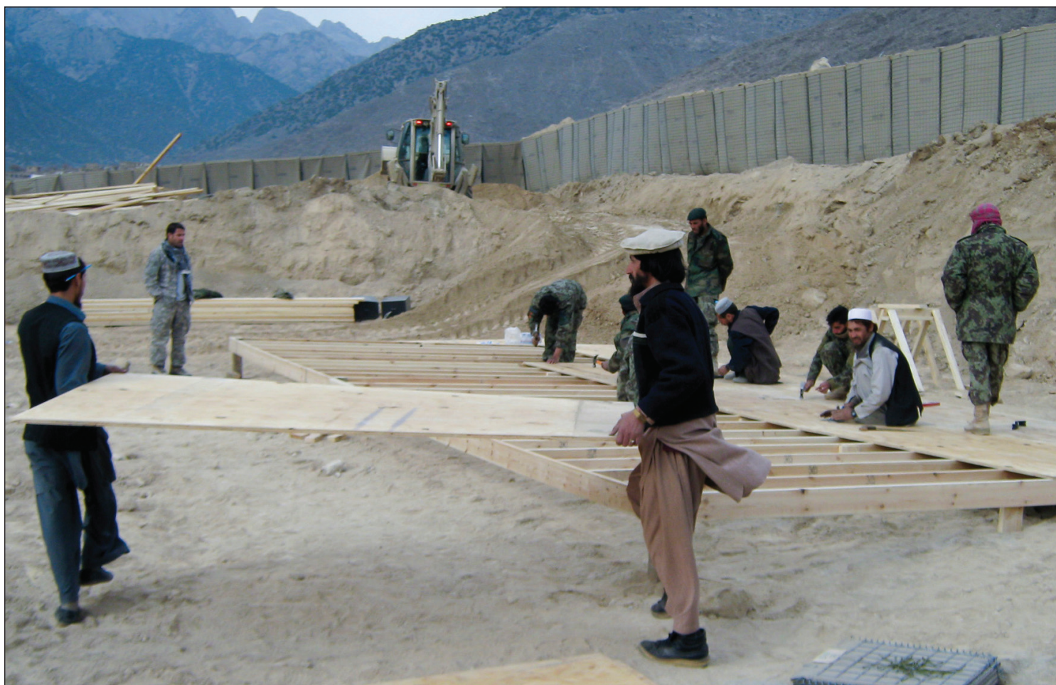
Afghan carpenters carry a cut piece of plywood to be used as the floor of a building at an Afghan National Army combat outpost just outside of Dawlat Shah District, Laghman Province. This is the first COP designed and built by the ANA with only minimal assistance from Coalition Forces. (Photo courtesy of TF Thunderbird, PAO)
