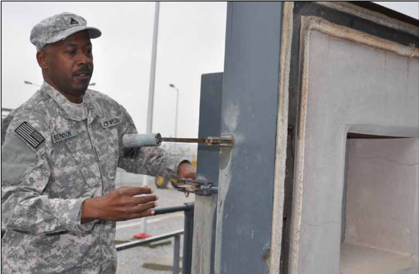
Construction representative Keith Benson opens a heavy door to one of the van-sized burn chambers at the new trash disposal plant at Bagram Airfield on Nov. 8. When in use, the chambers reach 1,800 degrees Fahrenheit.
