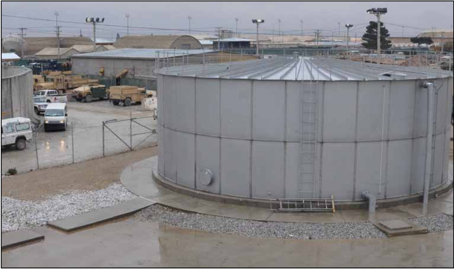
The $41.7 million water infrastructure upgrade features nine 211,000-gallon water storage tanks.
