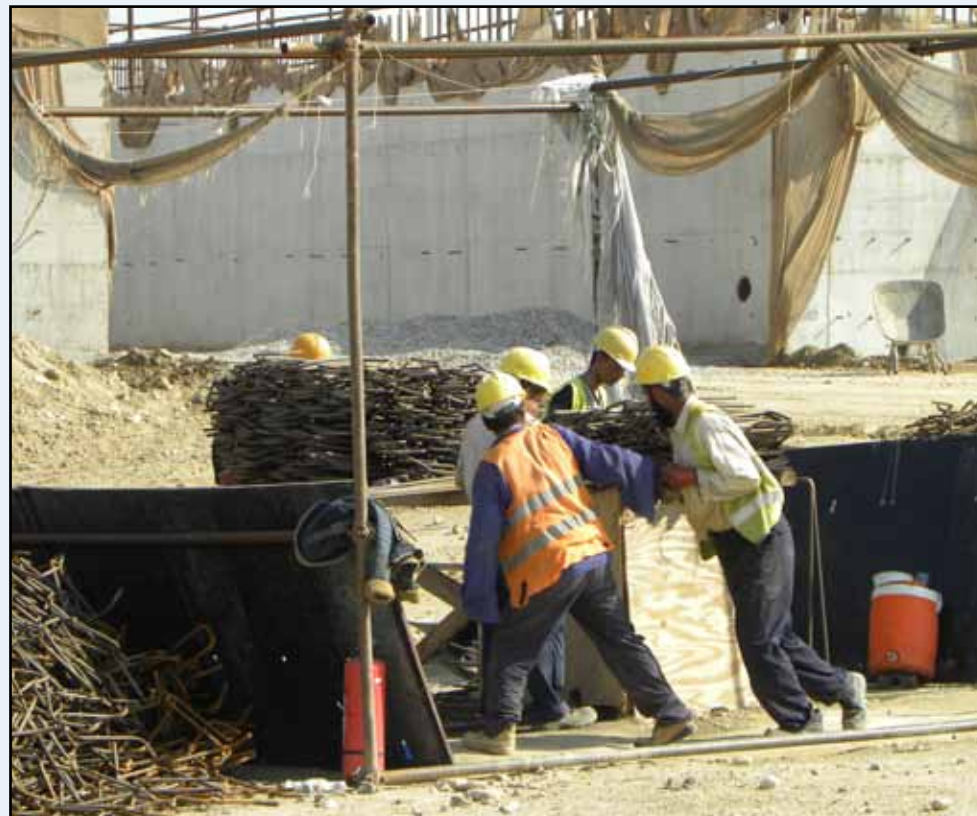
Construction workers shape rebar used to build the ammunition bunkers.
