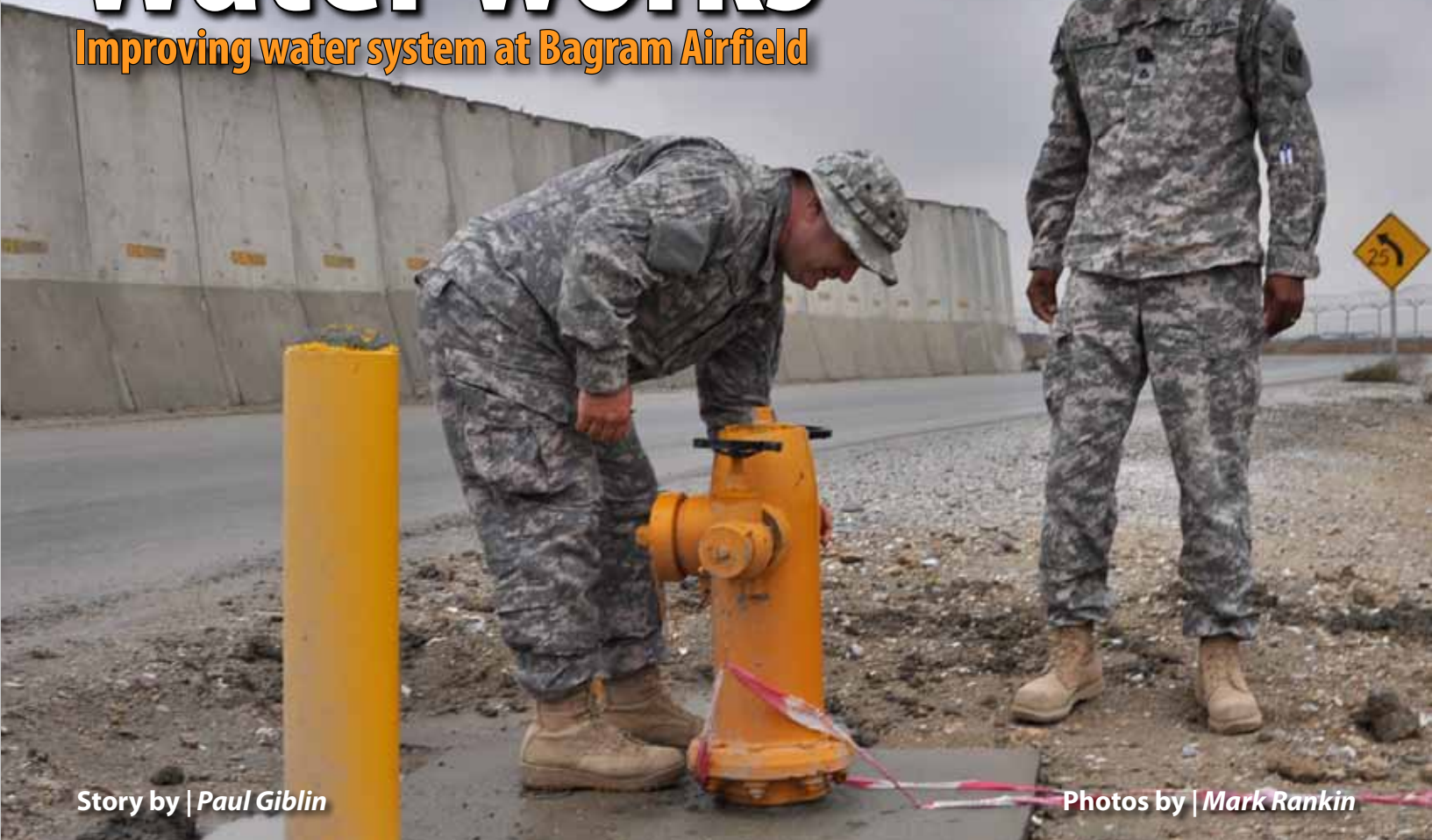
Construction representatives David Hoopengartner (left) and Keith Benson check the pressure at one of 284 fire hydrants at Bagram Airfield on Nov. 9.
