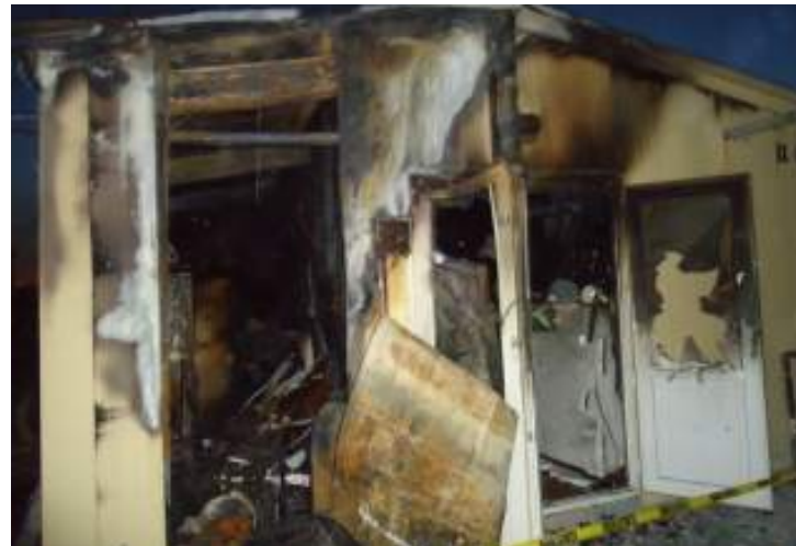
Living quarters destroyed in a fire caused by a non-approved power strip.
