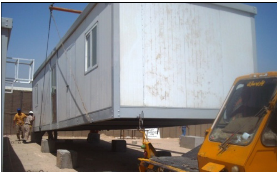
Setting a CHU in place during the buildup.
