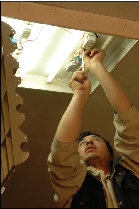
(Top) An Afghan electrician with the Haji Azizullah Mohammad Construction Company runs wire for new perimeter security lights on an Afghan National Police compound in Bazarak District, Afghanistan. The company was contracted by the Panjshir Embedded Training Team to install electrical wiring and lighting at two ANP facilities. (Above right) An Afghan electrician with the Haji Azizullah Mohammad Construction Company makes the final adjustments to a light fixture in the Dara District Afghan National Police compound.
