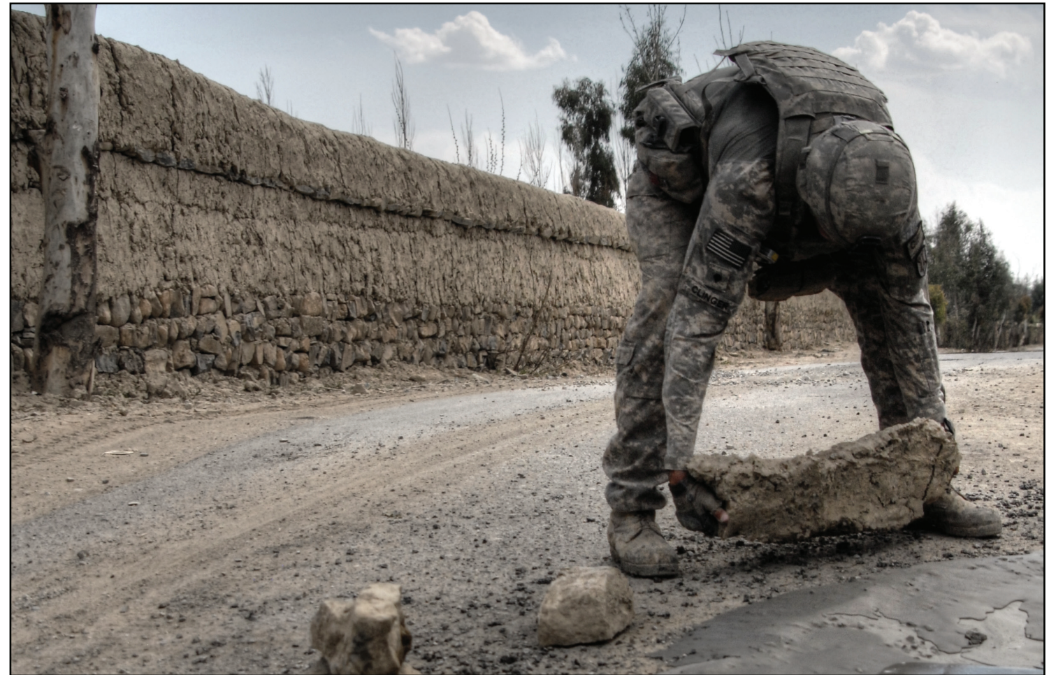
U.S. Army Spc. Daniel “Clinger” Vigil of Monticello, Utah, a combat engineer with 1st Platoon, 118th Sapper Company, sets rocks around a recently patched section of road outside of Yaqubi Village, Khowst Province, March 24. The placing of the rocks help to deter drivers from passing over the section of road and potentially damaging the fresh patchwork.
