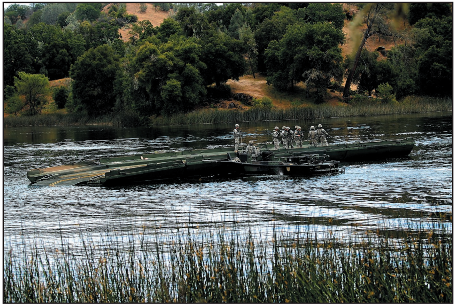
Members of the 671st Engineer Company stand atop their completed Improved Ribbon Bridge in Hughes Reservoir. The unit was in and out in less than seven hours.
