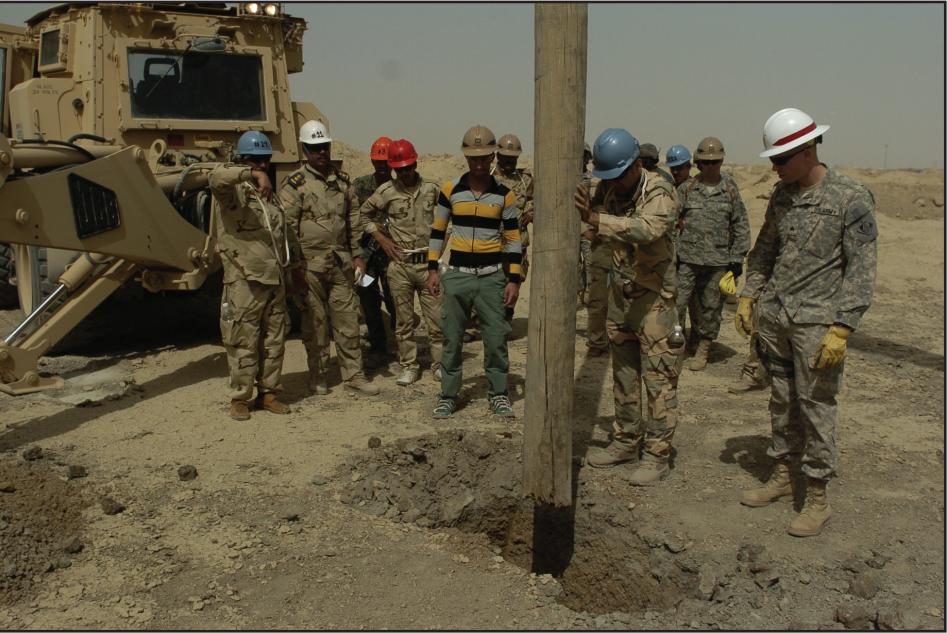
Sgt. Jessie Correia (right), a power line distribution specialist and power academy instructor, Co. D, 249th Engineer Battalion, assists Iraqi students on basic pole setting procedures and communicating with the operator as part of hands-on training April 17 at the Ali Air Base power training facility in Iraq.
