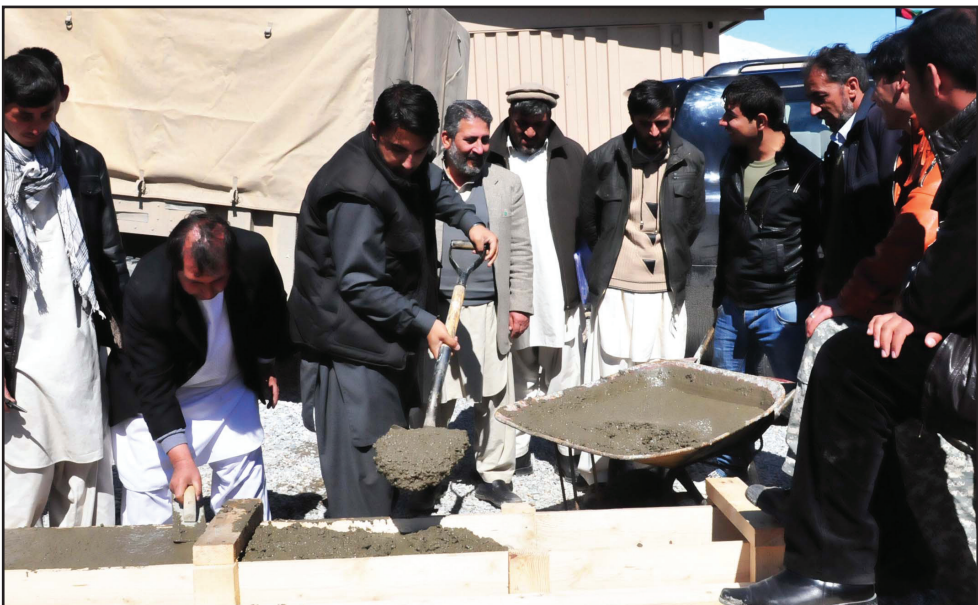
(Above) Panjshir Provincial Reconstruction Team's hands-on construction workshop attendees lay concrete in a ring beam during the "practical" portion of the workshop. The concrete will be broken later on to show the different results of using improper techniques compared to methods taught during the workshop (Below) During Panjshir Provincial Reconstruction Team's construction workshop March 8, attendees prepare to test a batch of concrete for its workability and water content before the concrete is to be used.
