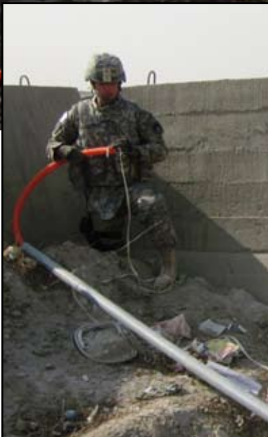
Right, Air Force Senior Airmen Bryant Laris and Derek Sams, both cable/antenna journeyman, pull off enough inner-duct for installation into an underground communication system. The inner-duct is used to protect Fiber Optic Cable from being damaged during installation.
