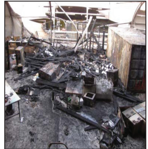
The debris of a burned-down section of a tent remains visible after faulty electrical wiring shorted out.
