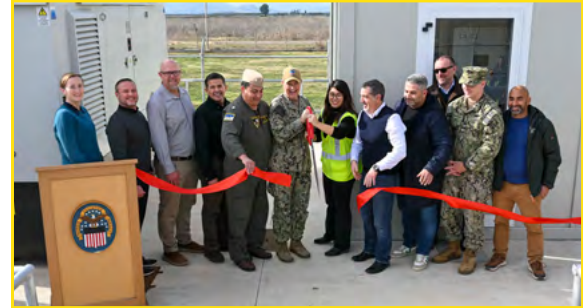
The Defense Logistics Agency Distribution Sigonella, Italy, unveils its new solar array and Battery Energy Storage System with a ribbon-cutting ceremony, January 15. The microgrid teams with NAVFAC EXWC and the Naval Postgraduate School were part of this years-long project.
