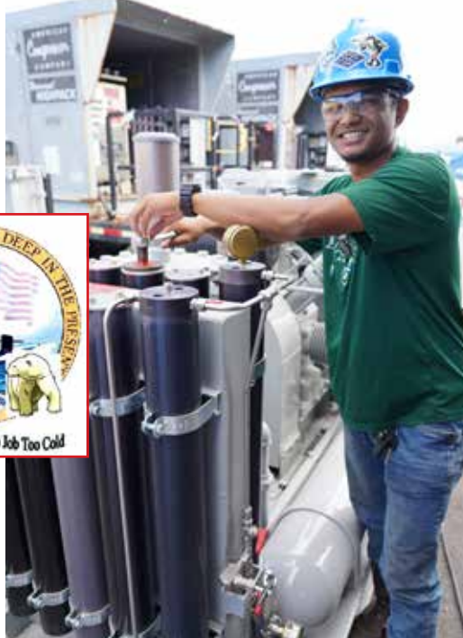
Shop 06 Production Machinery Maintenance Helper Reese Echavaria performs operator checks prior to starting a Temporary High Pressure Air Compressor (HPAC) which supports air charges to submarines.
