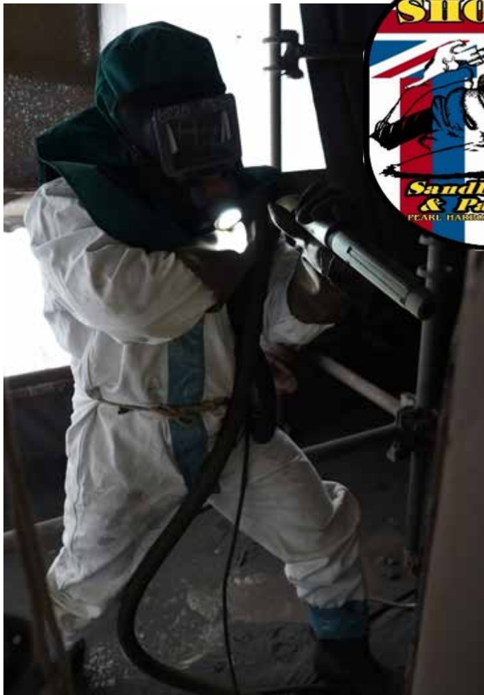
Shop 71 Painter/Blaster Work Leader, Jesse “Liko” Kruse, blasts a mockup of a submarines hull in preparation of USS Minnesota (SSN 783).
