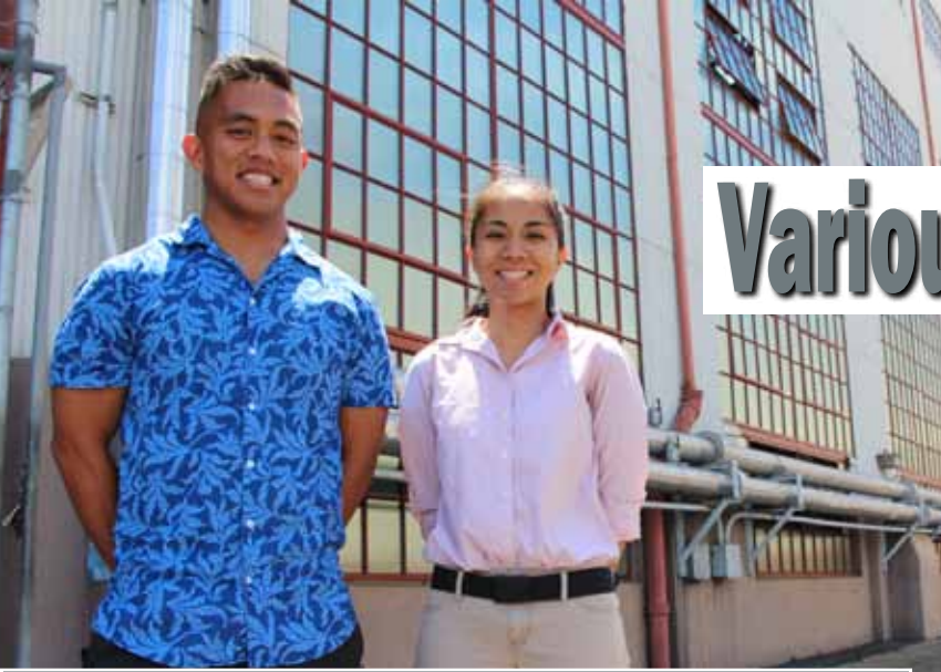
C930 Machinist Christian Smith and Code 981 Facilities Engineer Jhadyne Felipe are pictured at Building 67 which is currently undergoing window replacements to fix outstanding deficiencies while maintaining the historical appearance of the facility.
