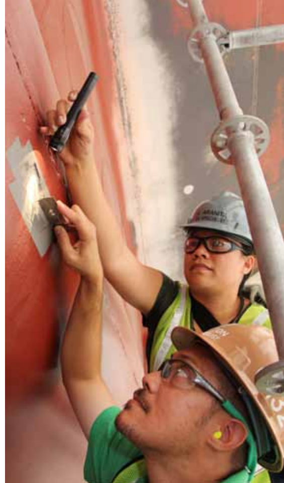
Code 132 Quality Assurance Specialists Lawrence Patton and Kai Aranita, provide government Nondestructive Testing (NDT) oversight of contractor work on the external stern tube of the USS Halsey (DDG 97.)
